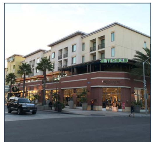
The use of quality materials and finishes in building design can enhance the identity of the corridor.
