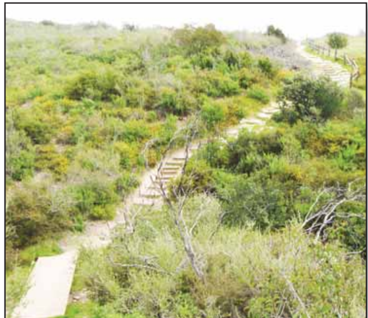
An excessively steep and eroding section of trail recommended for rerouting (FM-R7)
