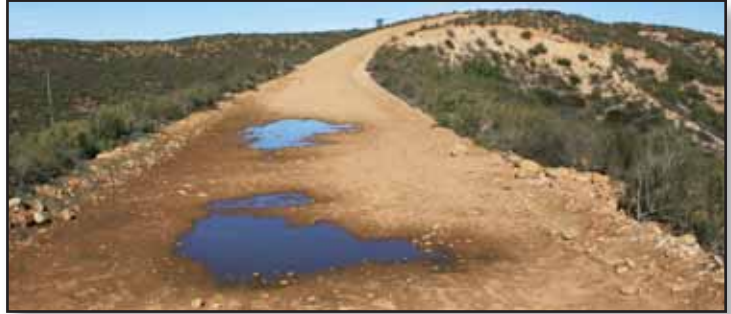
Utility road maintenance grading has created berms along the edges preventing proper drainage
