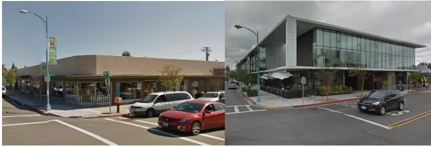
Figure 8. North Park site before and after redevelopment
