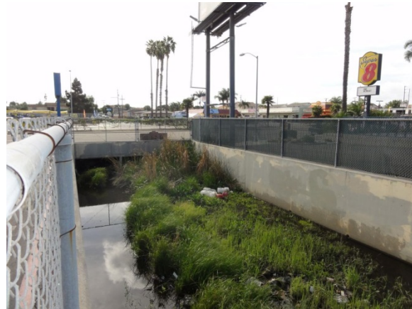
The downstream side of the Palm Avenue triple RCB culvert, Reach 1b facing upstream.
