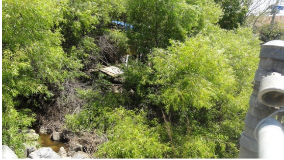
The downstream portion of Reach 5.
