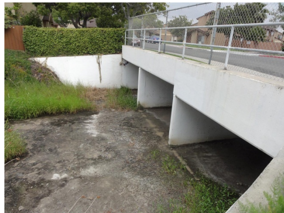
The upstream side of the Cerrissa Court triple RCB culvert, Reach 4.
