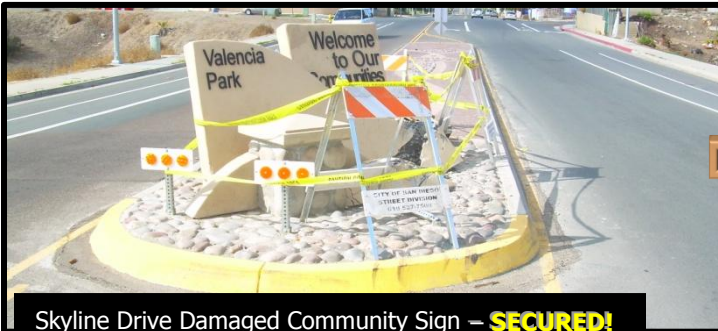
Skyline Drive Damaged Community Sign – SECURED!
