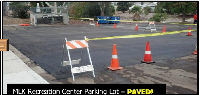
MLK Recreation Center Parking Lot – PAVED!
