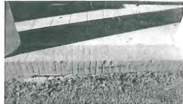
Inappropriate painted masonry edge which was originally left unpainted at Building 10. Photograph courtesy of Architect Milford Wayne Donaldson, FATA, January 10, 2000.
