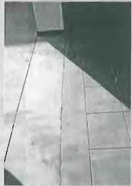
Inappropriate new concrete substituted for original masonry edge at arcade. Photograph courtesy of Architect Milford Wayne Donaldson, FAIA dated January 11, 2000.
