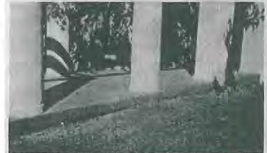
Painted brick banding found on the arcade walkways should be returned to the natural brick finish. Photograph courtesy of KTU+A, February 2000.
