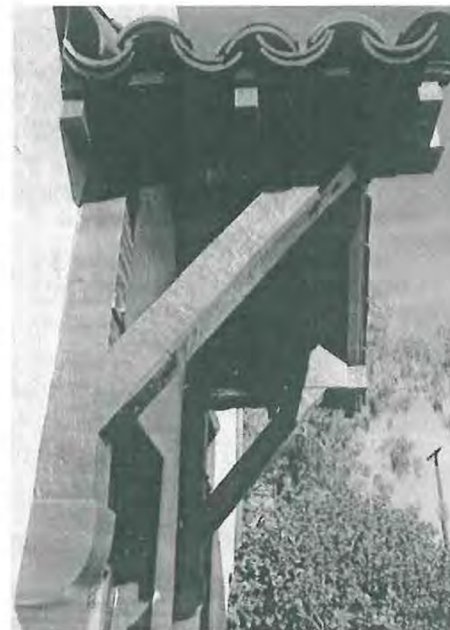
Several wood members are fastened by metal plates and bolts, but need to be seismically analyzed. Photograph courtesy of Architect Milford Wayne Donaldson, FAIA, January 10, 2000.
