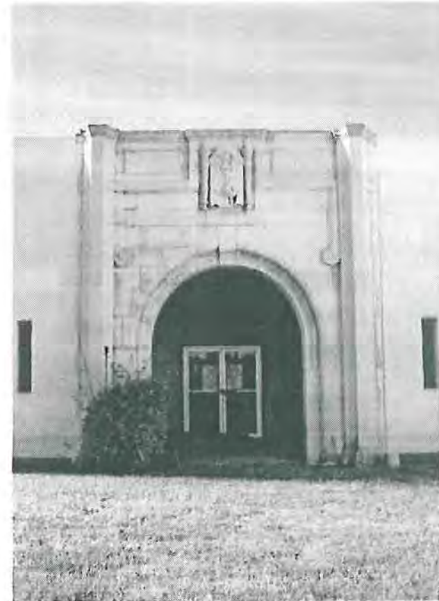
Entrance to the Mess Hall in Building 30. The historic doors have been removed and replaced with aluminum frame doors (this is not recommended). Photograph courtesy of Architect Milford Wayne Donaldson, FAIA, January 11, 2000.
