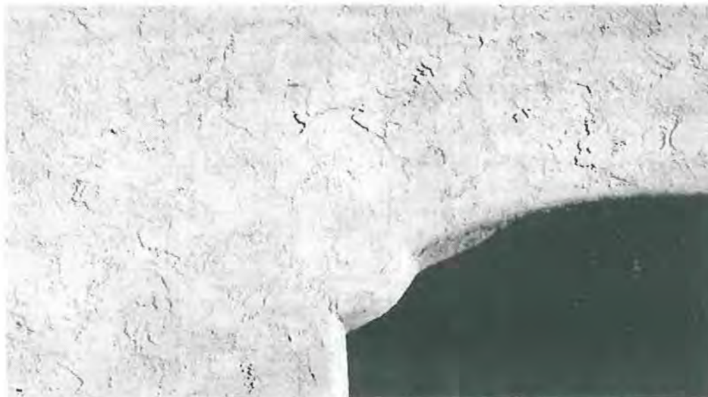
A heavy "skip trowel" stucco skim coating has been applied to Officer's Quarters "A" and has greatly changed the original adobe style finish. Photograph courtesy of Architect Milford Wayne Donaldson, FAIA, January 10, 2000.
