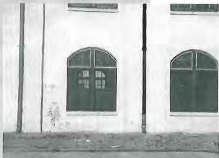
Stucco texture and color chipping in several buildings. Photograph courtesy of Architect Milford Wayne Donaldson, FAIA, January 27, 2000.
