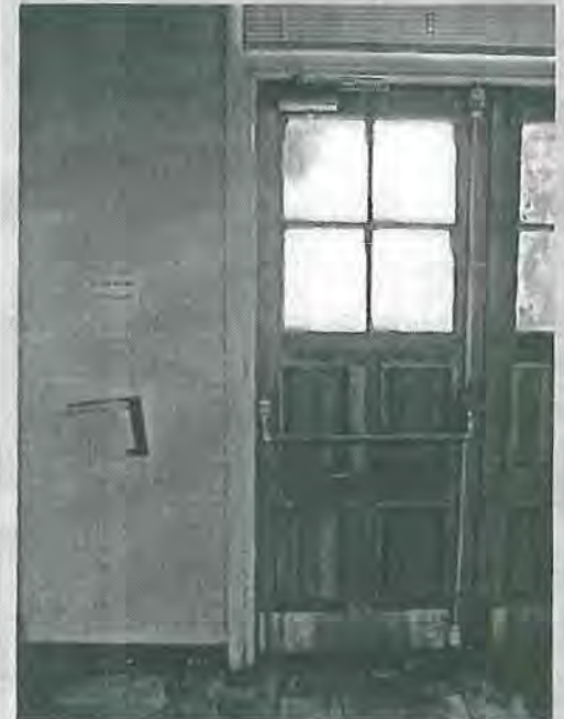
Several exit doors have been retrofitted with panic hardware; however exit signs have not been installed. All exit doors should have illuminated exit signs. Photograph courtesy of Architect Milford Wayne Donaldson, FAIA, February 2000.
