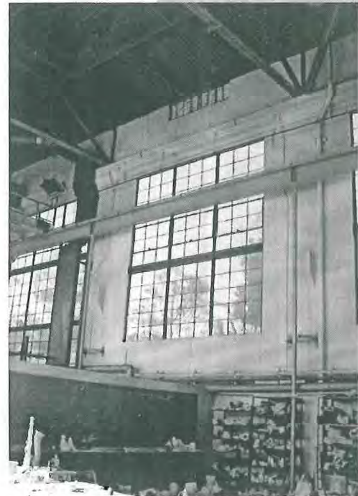
Exposed conduit and other mechanical systems in industrial spaces are appropriate. Photograph courtesy of Architect Milford Wayne Donaldson, FAIA, December 21, 1999.
