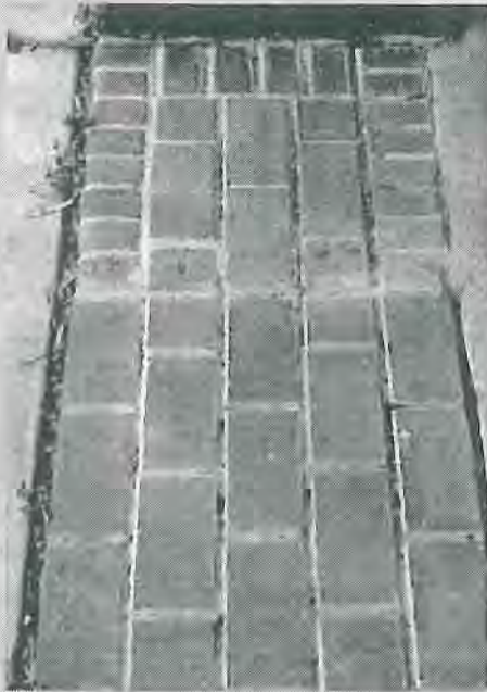
Inappropriate patch with modern brick not matching original pattern at Building 30. Photograph courtesy of Architect Milford Wayne Donaldson, FAIA, January 11, 2000.
