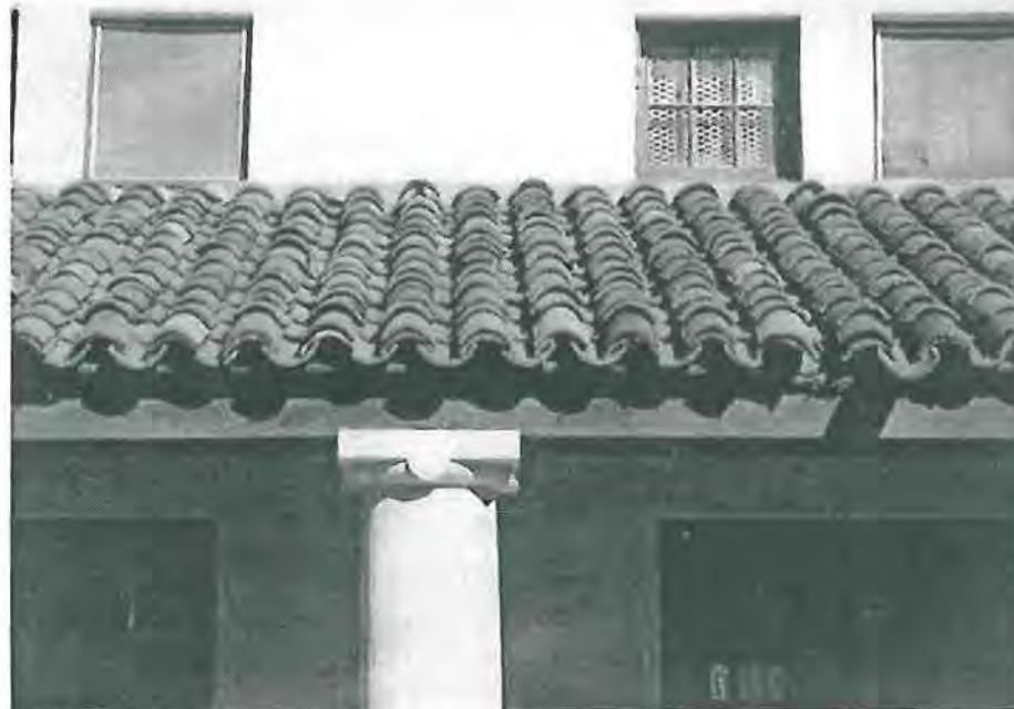
Original barrel tile roof at the rear facade of Building 25. Photograph courtesy of Architect Milford Wayne Donaldson, FAIA, January 4, 2000.
