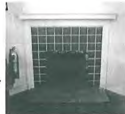
Fireplaces with undampened chimneys are a major source of heat loss. Nonfunctional chimneys should be covered by removable caps. Photograph courtesy of Architect Milford Wayne Donaldson, FAIA, December 21, 1999.
