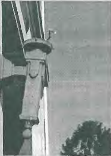
The original light fixture base is still present at Building 8, the Fire Station. The fixture should be restored to its original condition. Photograph courtesy of Architect Milford Wayne Donaldson, FAIA, January 11, 2000.
