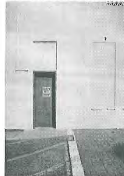
The building reveals an altered window that is now a door. There is clear evidence of the original window style form, materials, and color. Reconstruction of the altered window is appropriate. Photograph courtesy of Architect Milford Wayne Donaldson, FAIA, January 10, 2000.
