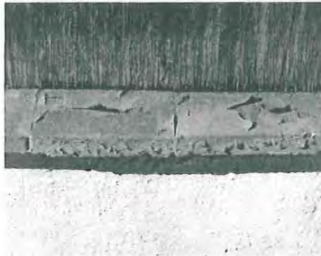
Inappropriate paint and color applied to window sill tile. Photograph courtesy of Architect Milford Wayne Donaldson, FAIA, January 4, 2000.
