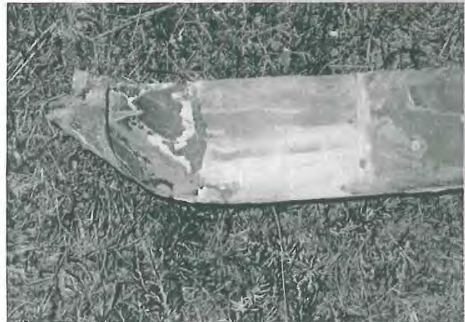
Copper downspout removed from Building 28 showing layers of paint. The downspouts were originally left unpainted. Photograph courtesy of Architect Milford Wayne Donaldson, FAIA, January 27, 2000.
