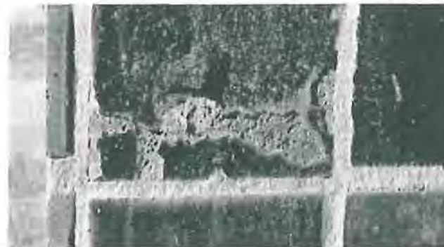
Glaze damage to terra cotta tile in the fountain near Building 20 and 21. Photograph courtesy of Architect Milford Wayne Donaldson, FAIA, January 10, 2000.
