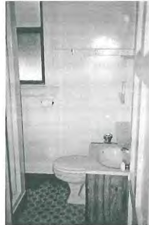
The original bathroom fixtures in the Officers' Quarters have been replaced with inappropriate plastic counters, sinks, toilets, and shower stalls. Photograph courtesy of Architect Milford Wayne Donaldson, FAIA, February 1995.
