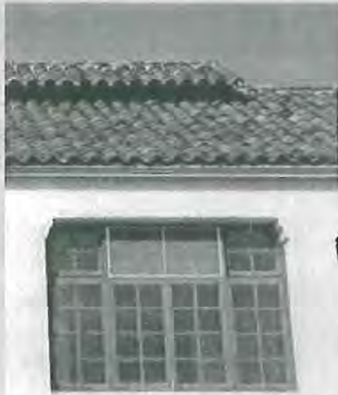
Wood framed raised roof for attic ventilation of barracks building. Note that the aluminum screen is not appropriate. Photograph courtesy of Architect Milford Wayne Donaldson, FAIA, January 11, 2000.
