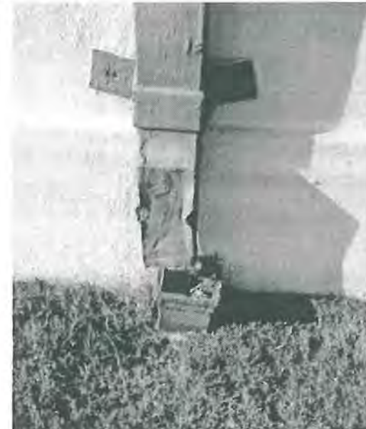
The downspout has been disconnected from the drain. The drain has become clogged with debris. This situation needs to be corrected to prevent water damage to the plaster walls and foundation. Photograph courtesy of Architect Milford Wayne Donaldson, FAIA, January 10, 2000.
