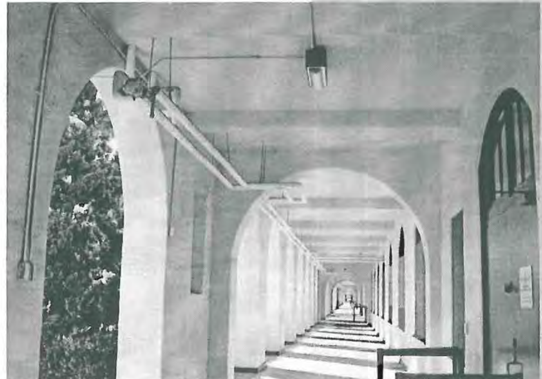
The exterior walls have exposed conduit and steam pipes that should have been installed away from the public view. Photograph courtesy of Architect Milford Wayne Donaldson, FAIA, December 21, 1999.
