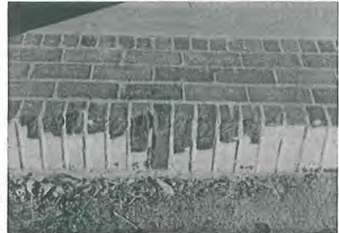
Bricks inappropriately painted and chipped at an arcade entrance. Photograph courtesy of Architect Milford Wayne Donaldson, FAIA, January 27, 2000.
