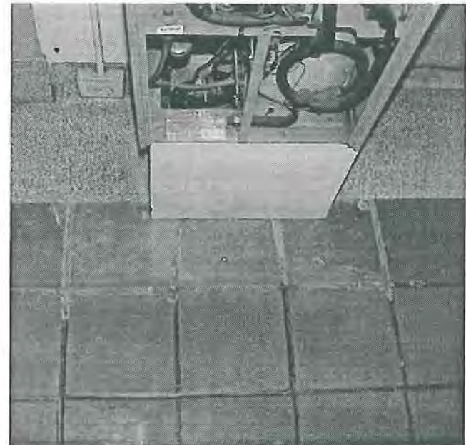
Leaking water cooler discoloring tile and mortar joints should be repaired to match original condition. Photograph courtesy of Architect Milford Wayne Donaldson, FAIA, February 2000.
