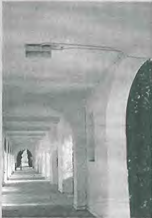
Original cast-in-place conduit has deteriorated and exposed conduit to service light fixture was installed over the archway. Attempts should be made to install new conduit to minimize visibility from public view. Photograph courtesy of Architect Milford Wayne Donaldson, FAIA, December 21, 1999.
