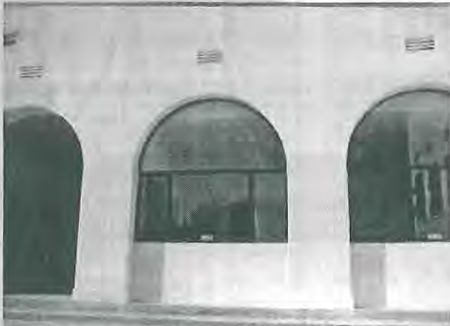
Some arches have been filled with modern aluminum windows, stucco infill, and dropped ceilings visible from the outside. These modifications are not in character with the historic buildings. Photograph courtesy of Architect Milford Wayne Donaldson, FAIA, January 11, 2000.
