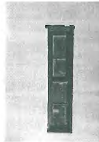
Historic wood window at Building 10, with small double-hung windows should be maintained and not replaced with aluminum windows. Photograph courtesy of Architect Milford Wayne Donaldson, FAIA, January 4, 2000.
