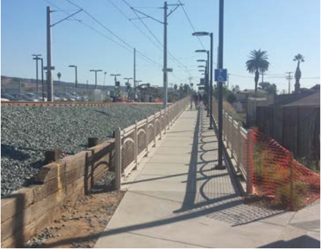
New pathway links Cottonwood Road to the Beyer Boulevard Trolley Station.
