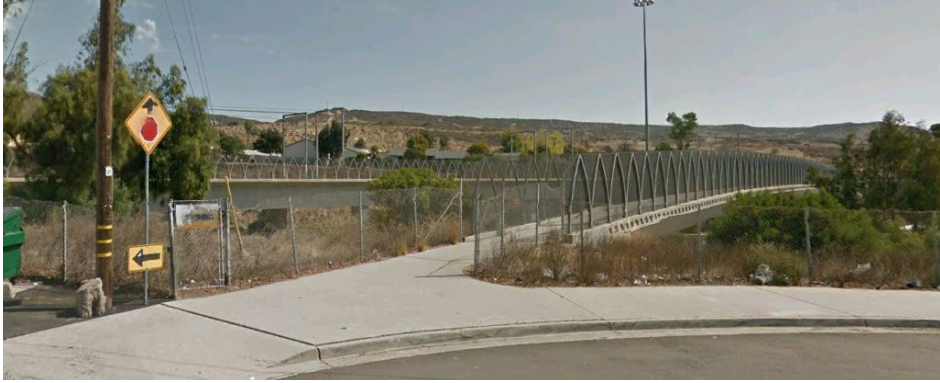
Existing condition at Olive Drive
