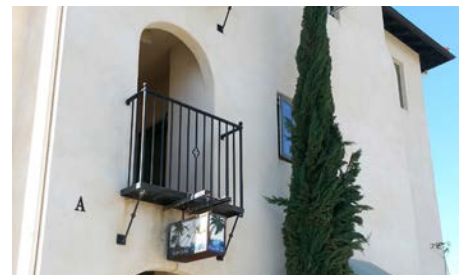
Windows, doors, and balconies add architectural elements while encouraging “eyes on the street”.
