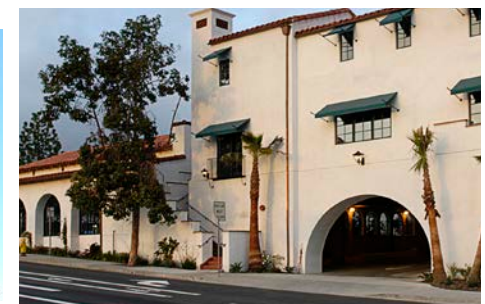
Examples of residential development with parking structures.
