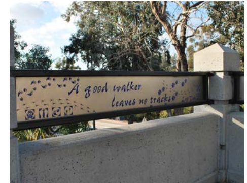
Public art incorporated into bridge railing.
