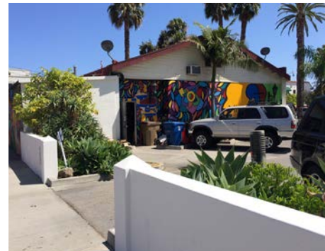
Low site walls and landscaping soften and screen parking.
