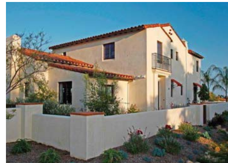
Semi-private courtyard enhances architecture.
