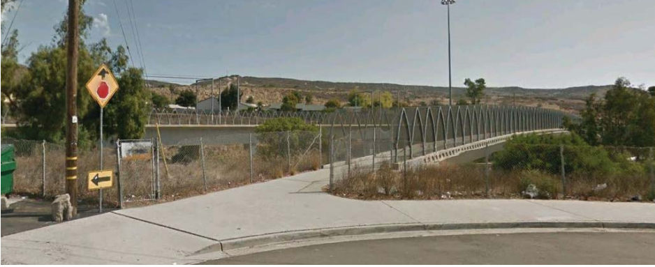
Existing condition at Olive Drive
