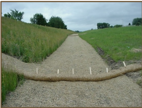
Hay wattles located at 15-foot intervals to stabilize slopes and control erosion.
