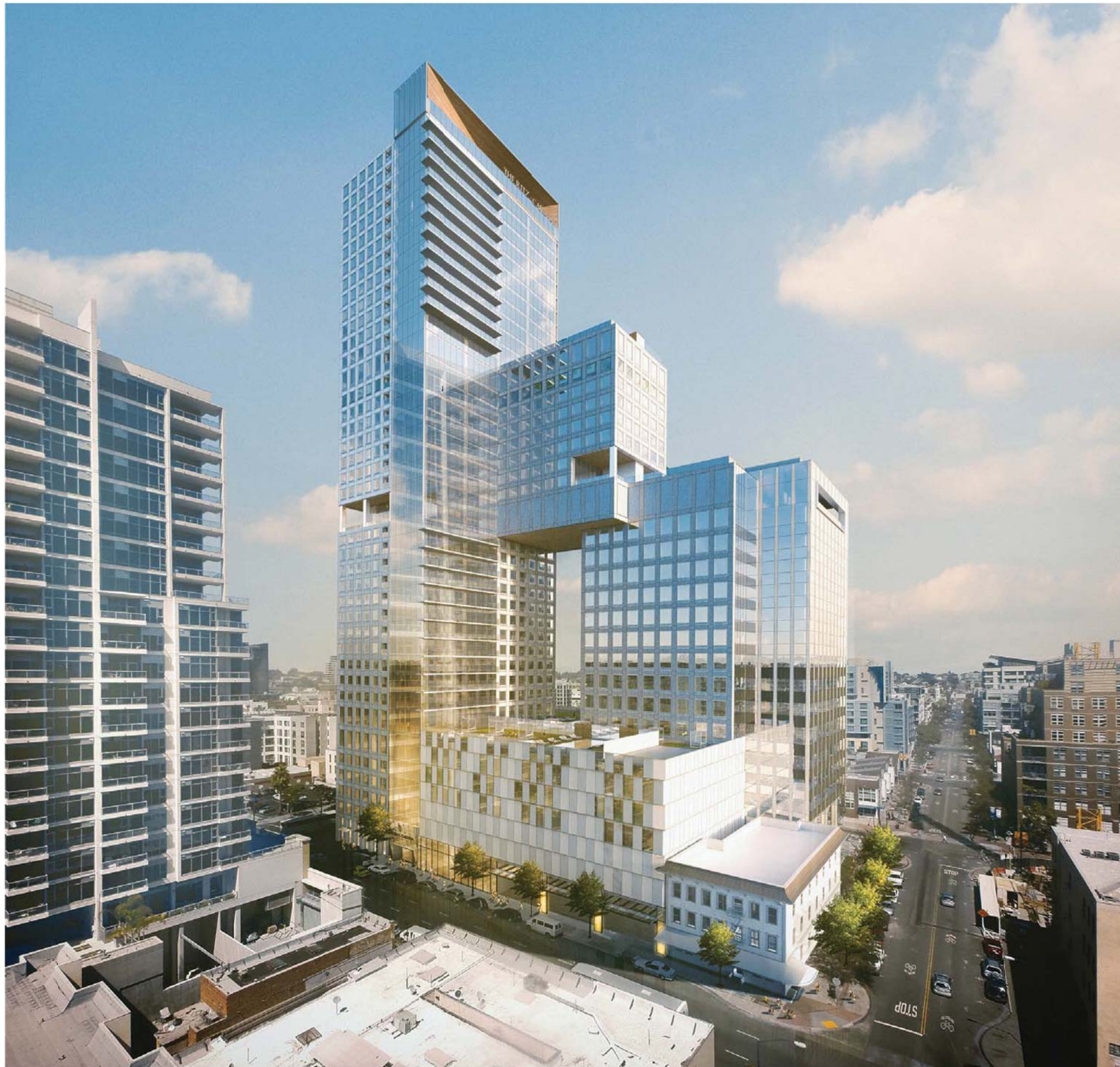
AERIAL VIEW FROM SOUTHWEST
