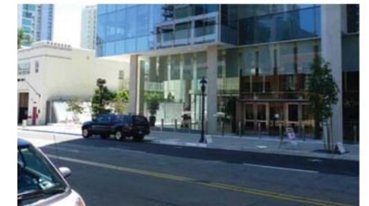
26. view southwest along 8th @ Island - Sempra tower base
