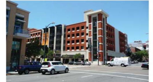
7. view northwest along Market - garage
