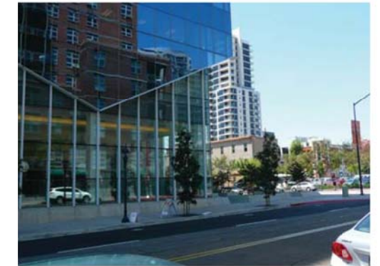
27. view northwest south along 8th - Sempra courtyard
