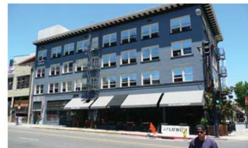
15. view northeast at Market @ 8th - apartments
