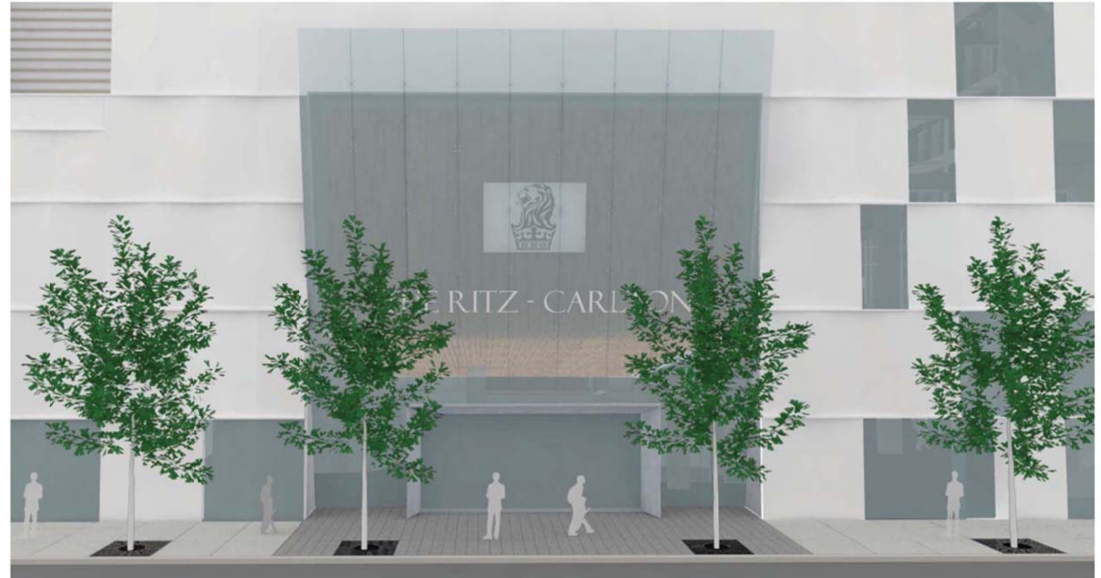
8TH AVENUE ENTRY
