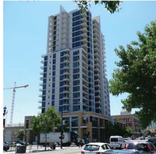
14. view west along Market @ 8th - Alta tower
