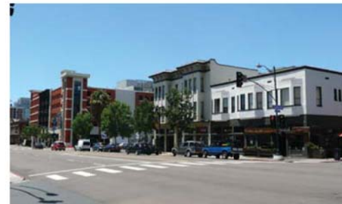
18. view northwest along Market @ 8th - apartments
