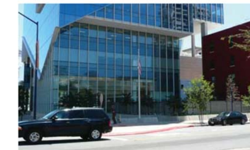
22. view south along Island @ 8th - Sempra tower
