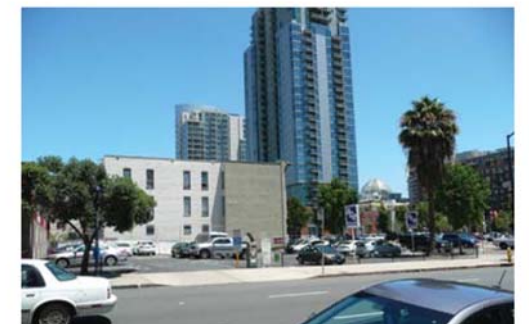
10. view east along 7th - parking lot
