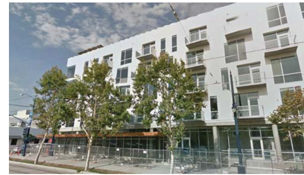
20. Views northeast along Park blvd. - Restaurant supply
