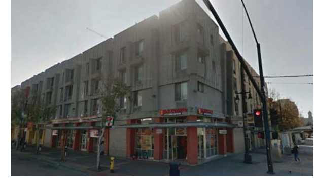
18. Views southwest along Park Blvd. - Residential
