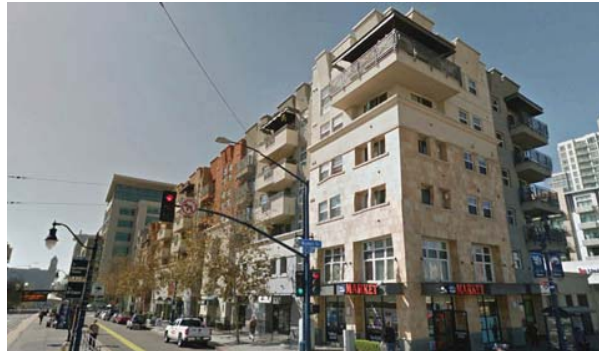
17. Views southwest along Market st. - Residential
