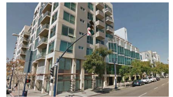
5. View west along 11th Ave. - Residential
