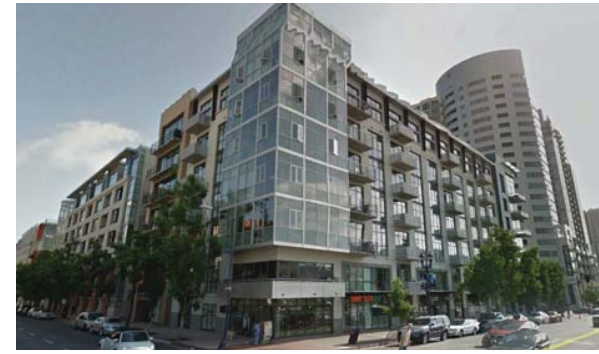
13. Views southwest along Market st. - Residential
