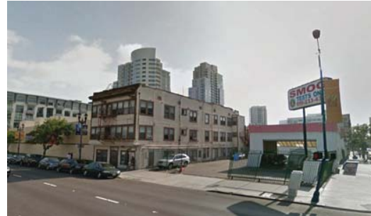
8. Views west along 11th Ave. - Smog Check
