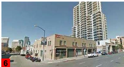
6 Street View: Corner of 7th & Island Ave looking at site
