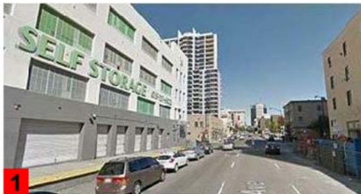
1 Street View: Looking North to Site
