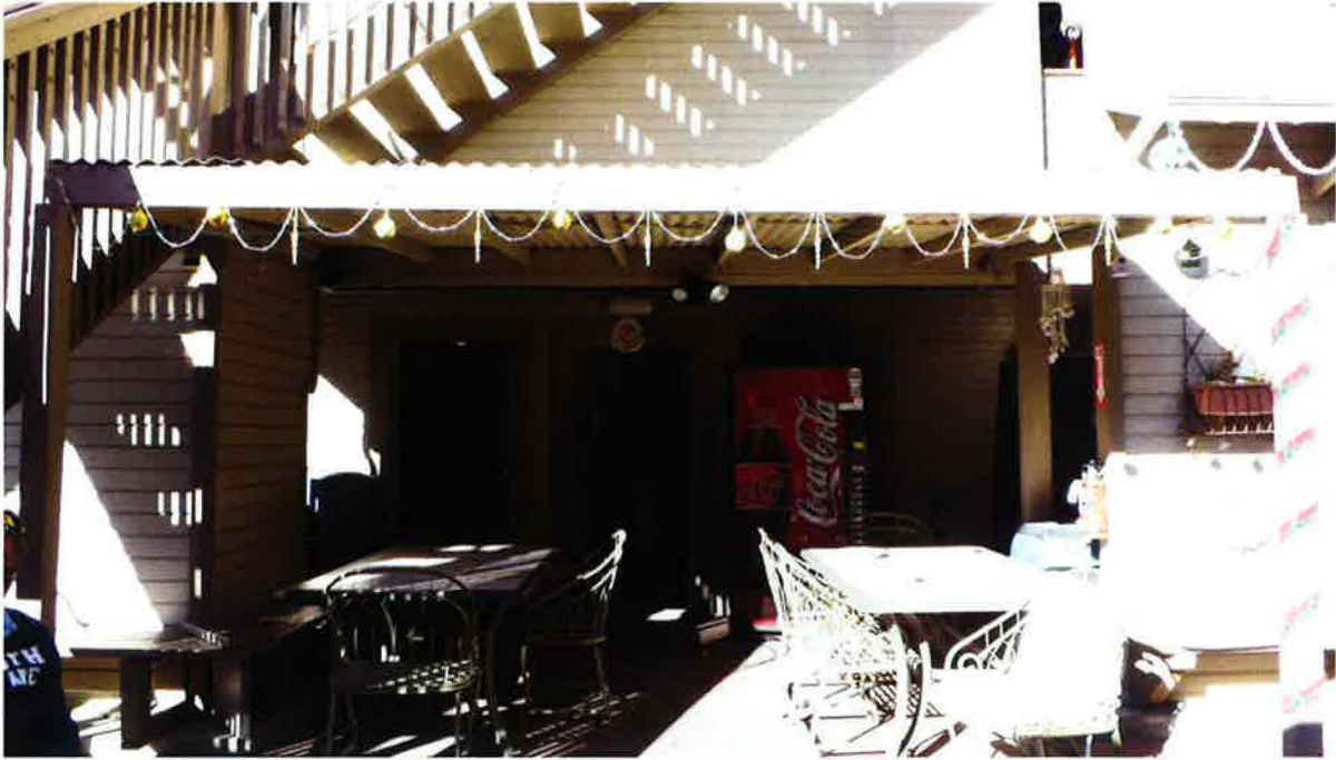
1425 C Street December 2015 Photograph #27 View North of ground level rear of the front building
