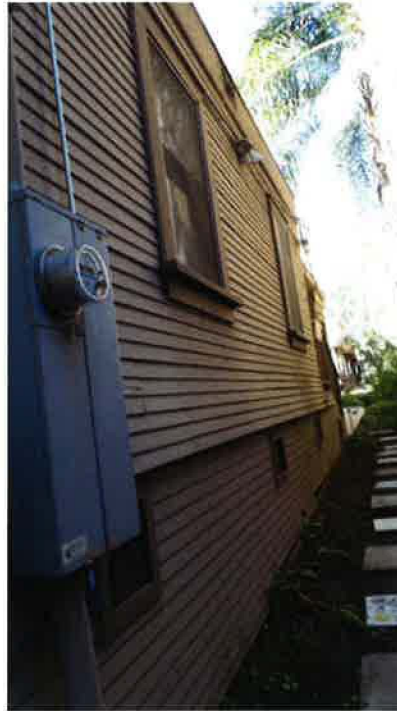
1425 C Street December 2015 Photograph #33 View North along East facade of rear building
