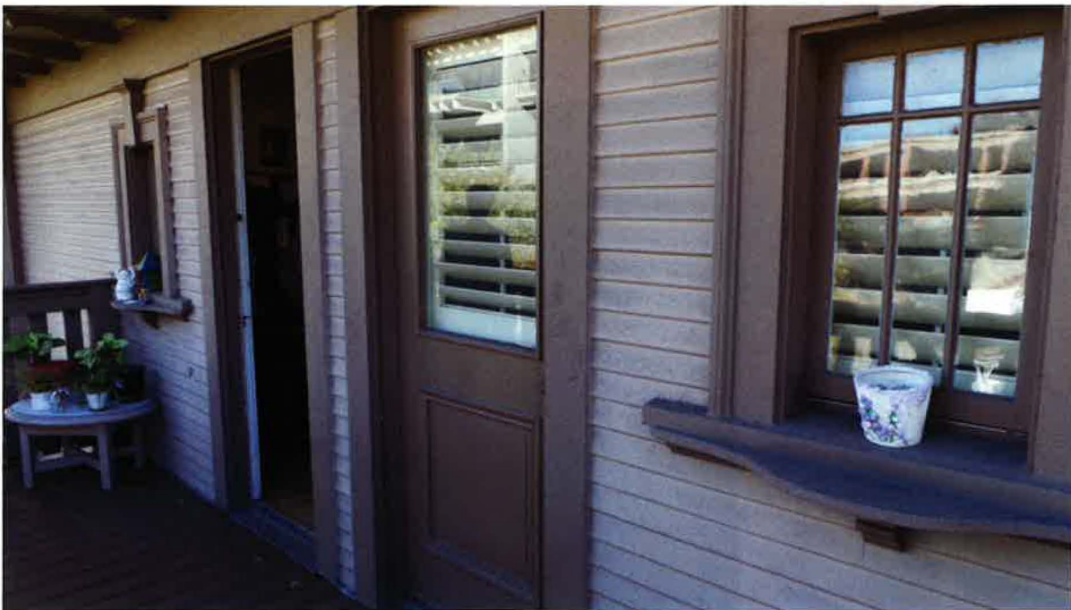
1425 C Street December 2015 Photograph #12 View Southeast second floor balcony, front building
