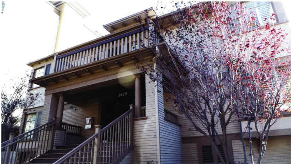
1425 C Street December 2015 Photograph #2 View Southeast of front façade
