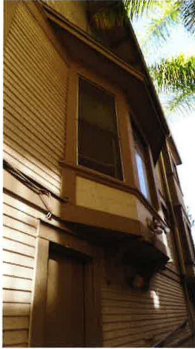
1425 C Street December 2015 Photograph #21 View North of East facade of the front building
