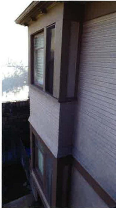
1425 C Street December 2015 Photograph #6 View east of projecting bay on front building
