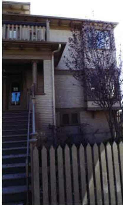
1425 C Street December 2015 Photograph #10 View South of front building west end
