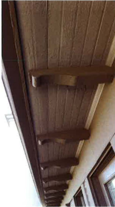
1425 C Street December 2015 Photograph #15 View East of second floor balcony detail
