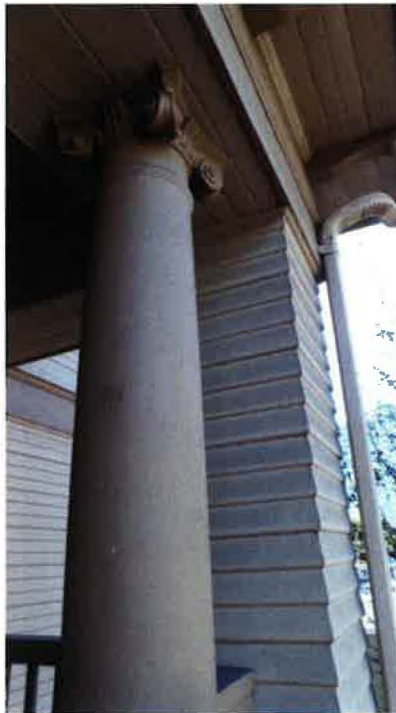
1425 C Street December 2015 Photograph #8 View Southwest of porch column
