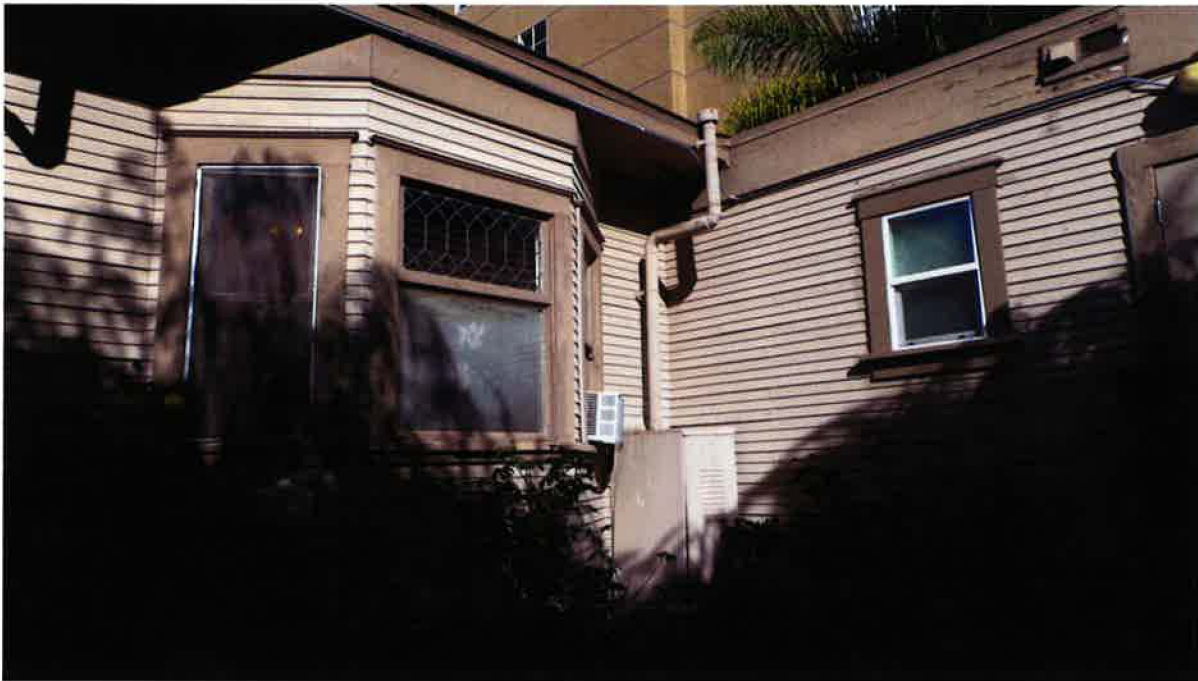
1425 C Street December 2015 Photograph #36 View Northeast of rear facade of rear building
