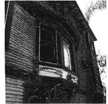
1 PHOTO: BAY WINDOW (EAST FACADE) HA 1 MARCH 2016
