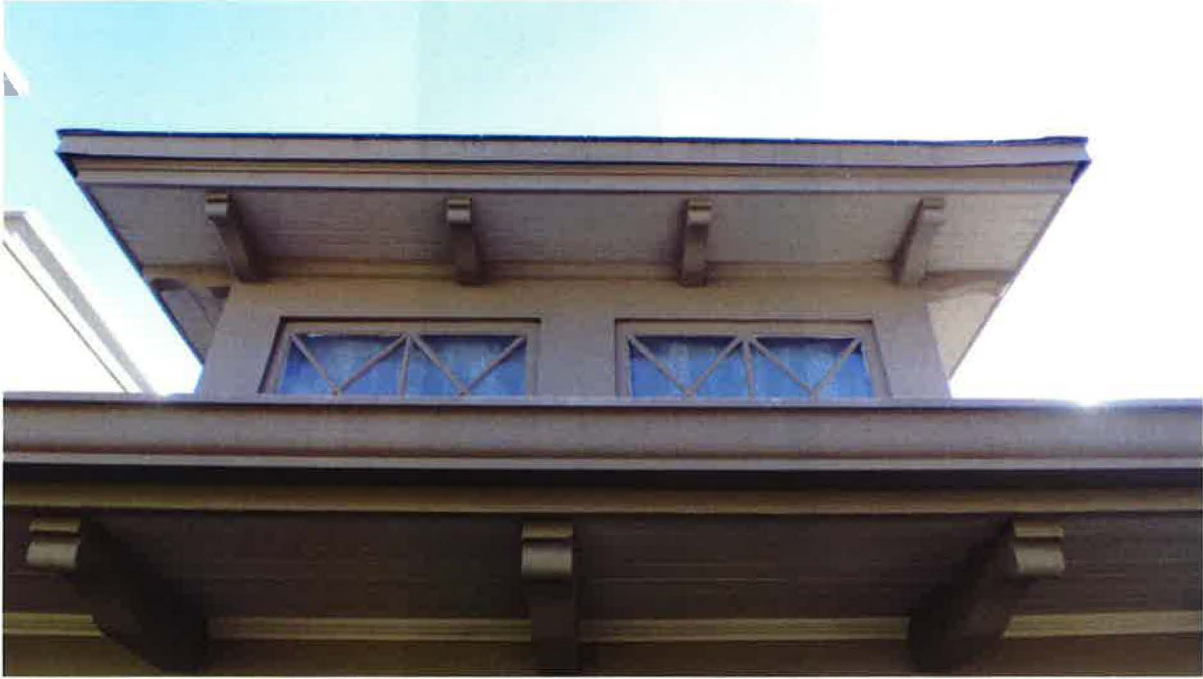
1425 C Street December 2015 Photograph #17 View of dormer above second floor balcony
