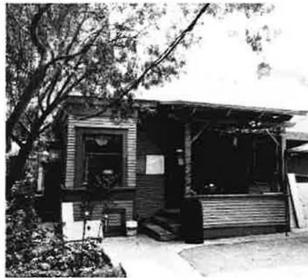
5 PHOTO: NORTH ENTRY PORCH HA 1 MARCH 2016
