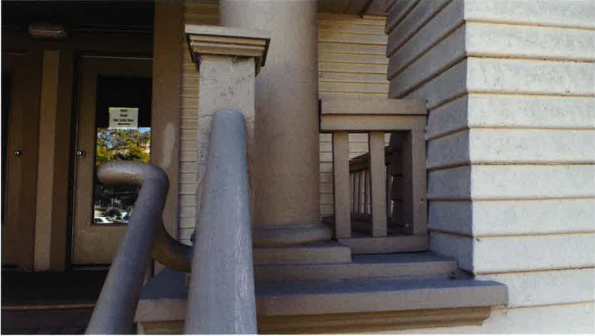
1425 C Street December 2015 Photograph #9 View North of porch column
