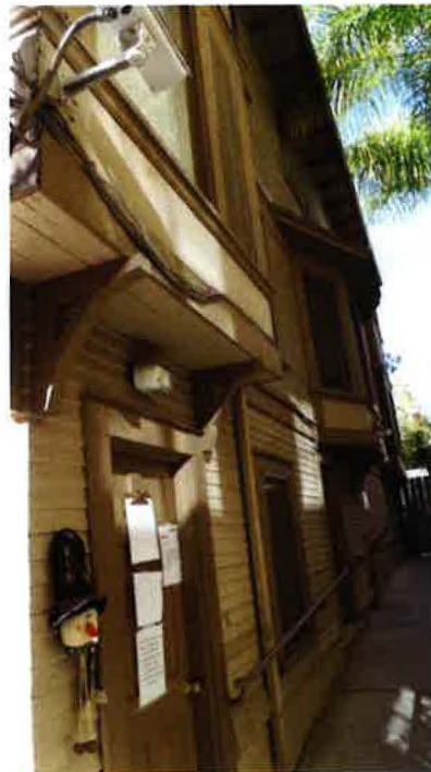
1425 C Street December 2015 Photograph #20 View North of East facade of the front building
