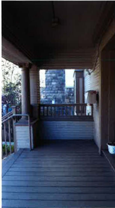
1425 C Street December 2015 Photograph #7 View East of first floor porch
