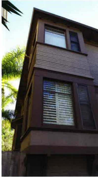
1425 C Street December 2015 Photograph #5 View South of front East corner of front facade
