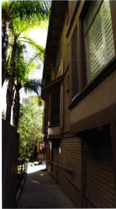
1425 C Street December 2015 Photograph #19 View South of East facade of front building
