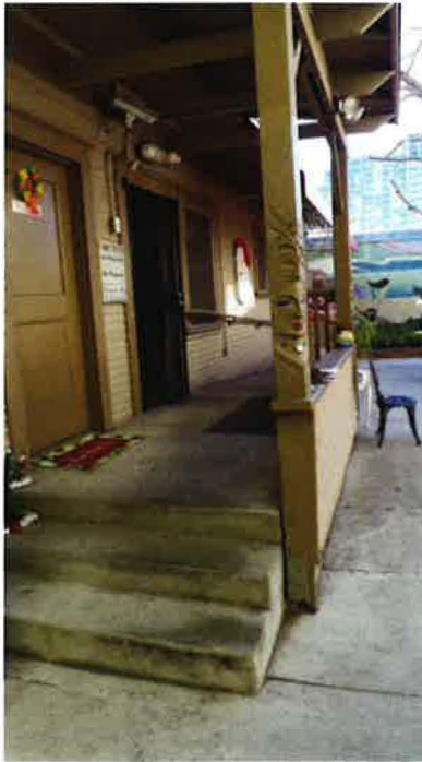
1425 C Street December 2015 Photograph #30 View West on North facade of rear building
