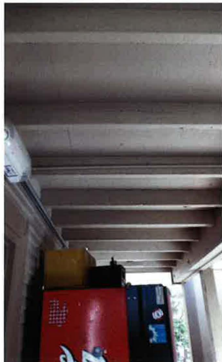
1425 C Street December 2015 Photograph #28 View East under porch rear of front building
