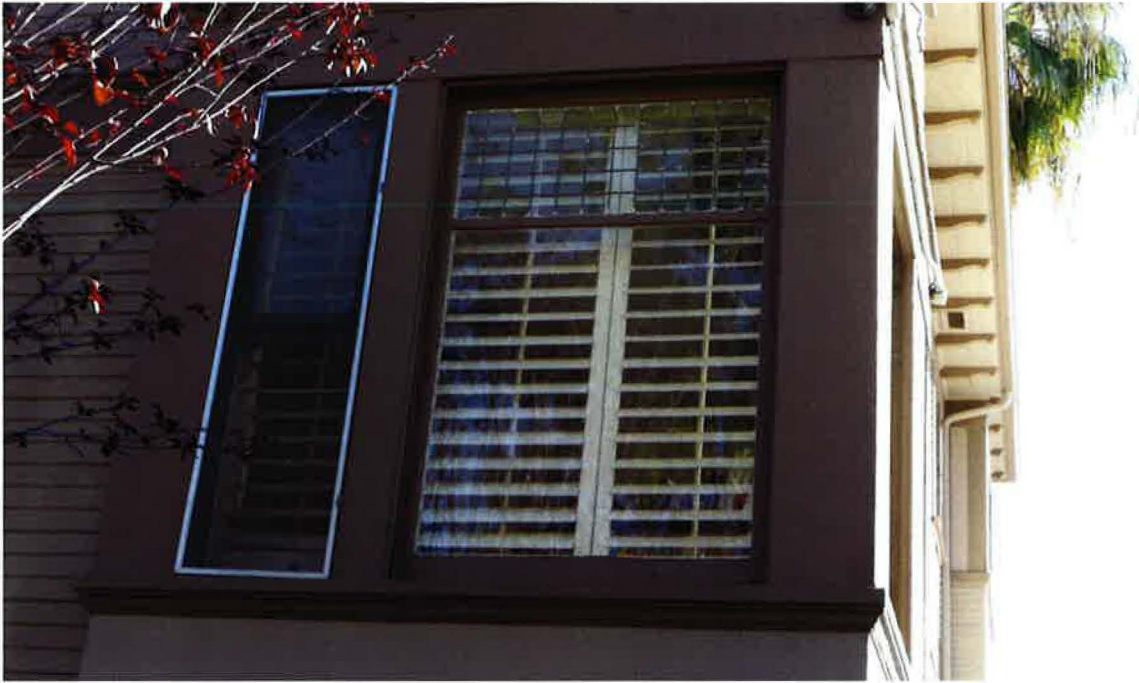
1425 C Street December 2015 Photograph #11 View North of windows front facade West end
