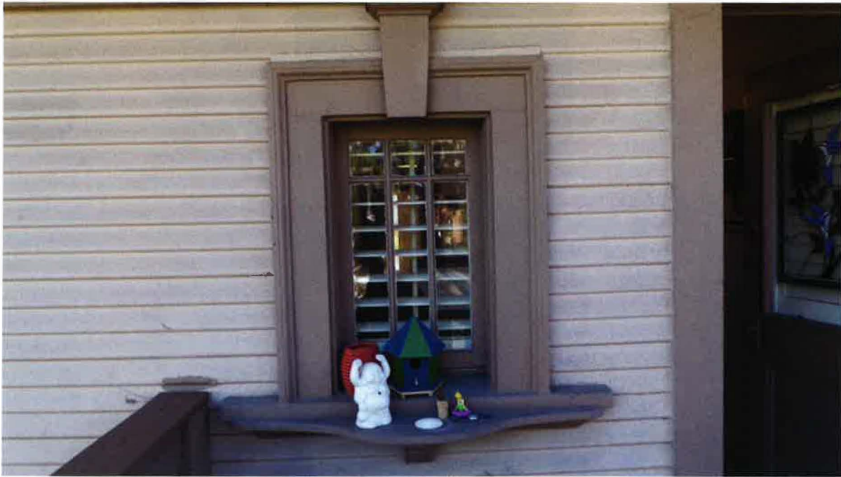
1425 C Street December 2015 Photograph #13 View South of windows and sill detail on second floor balcony, front building
