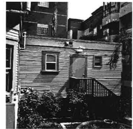
2 PHOTO: WEST FACADE HA 1 MARCH 2016
