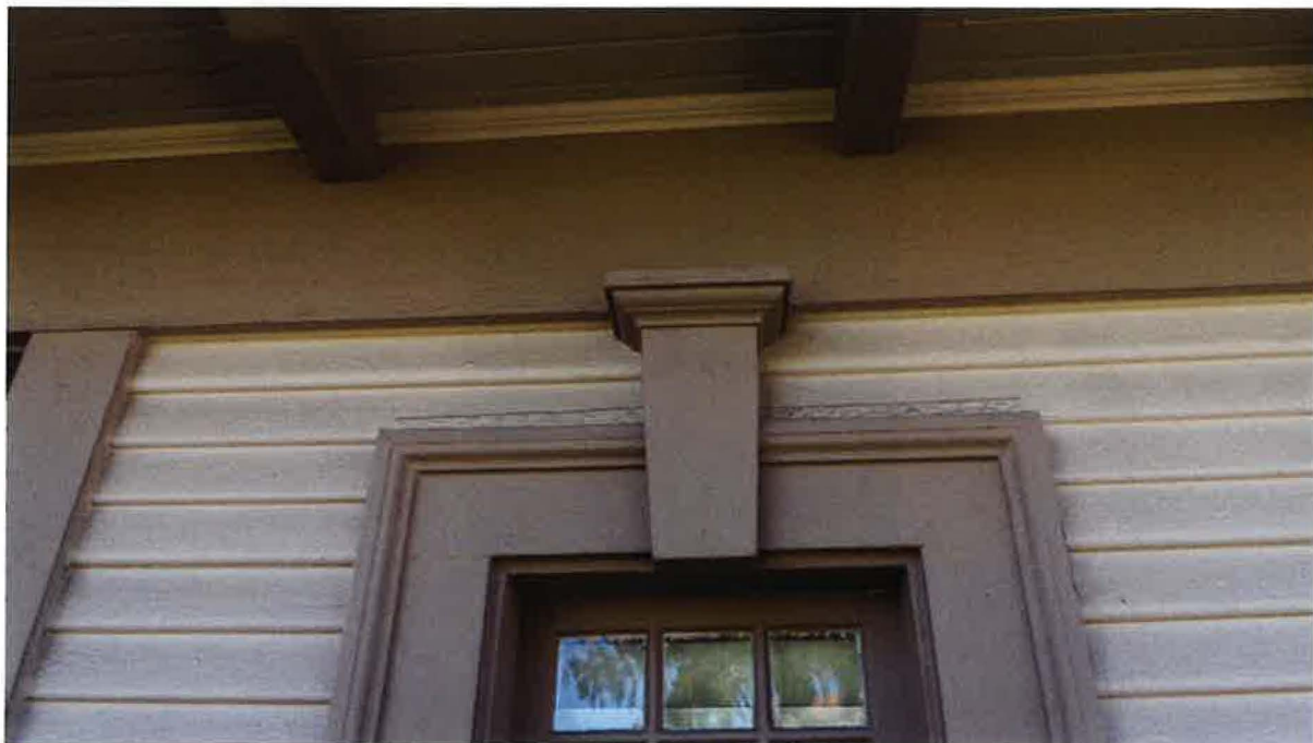
1425 C Street December 2015 Photograph #14 View of balcony detail
