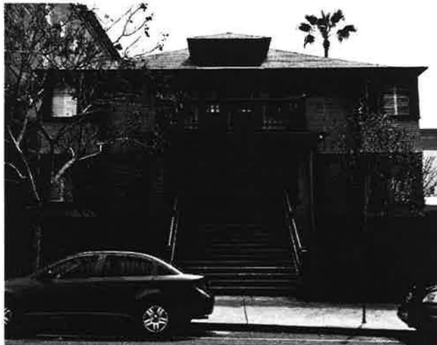
4 PHOTO: NORTH FACADE HA 1 MARCH 2016
