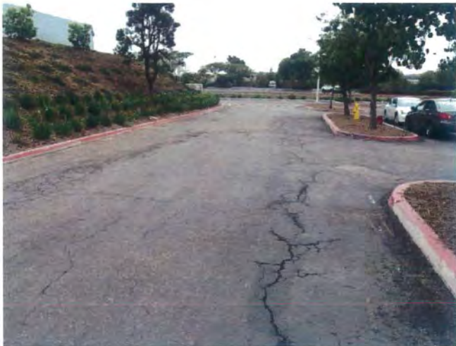
57 Failing pavement, fire lane, west of Central Plant
