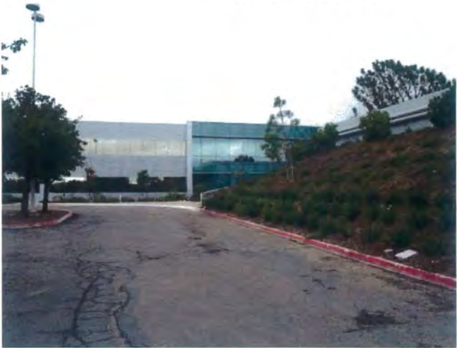
56 Failing pavement, fire lane, west of Central Plant
