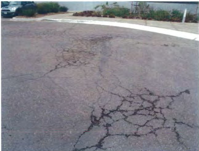
58 Failing pavement, fire lane, west of Central Plant
