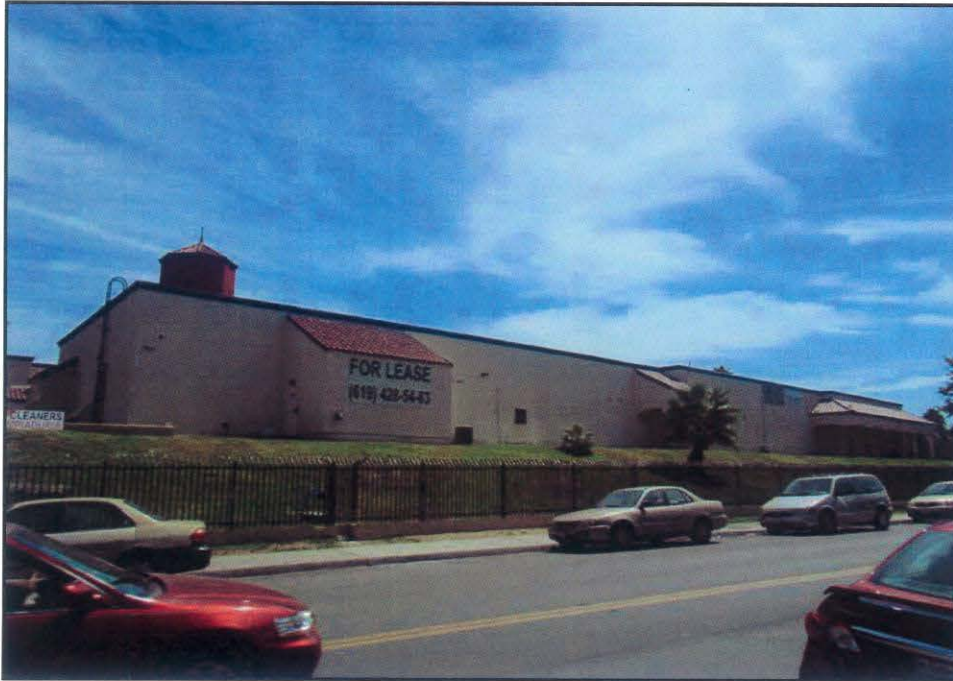
SITE PRIOR TO INSTALLATION
