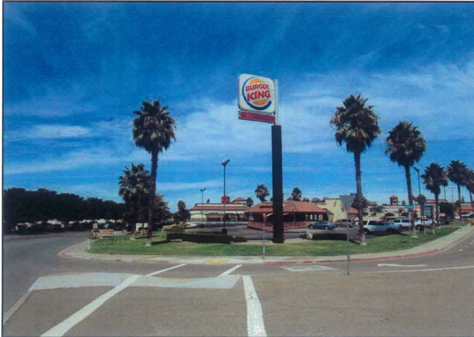
SITE PRIOR TO INSTALLATION
