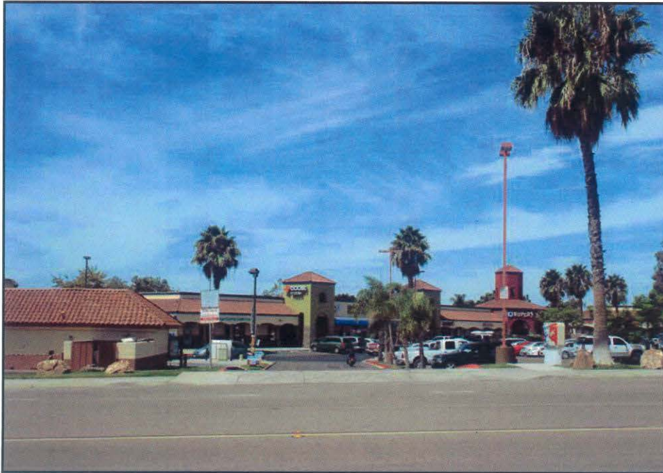
SITE PRIOR TO INSTALLATION
