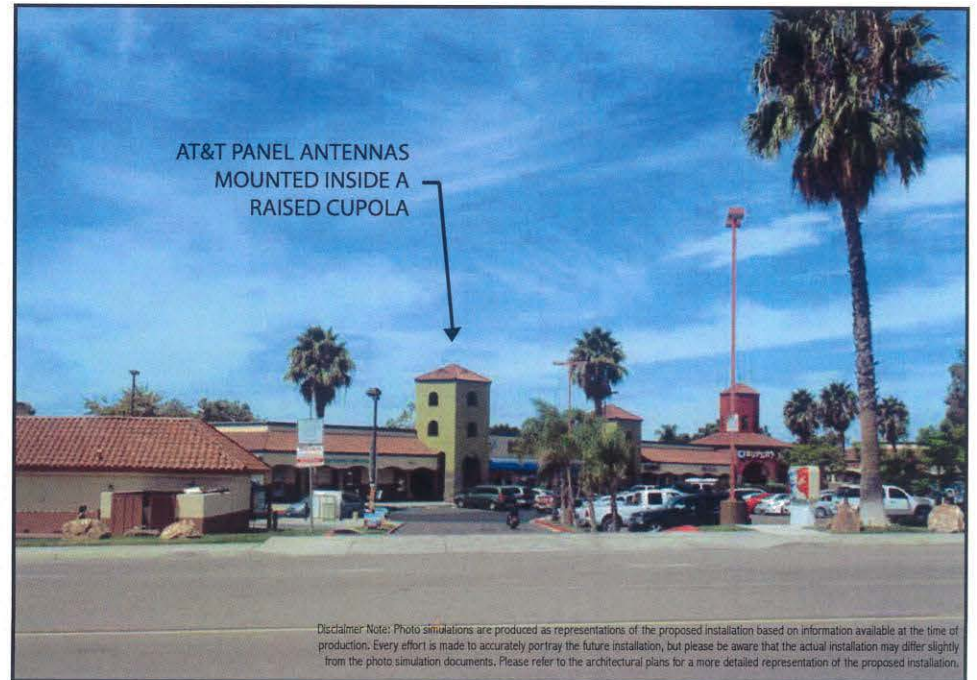
SITE AFTER INSTALLATION
