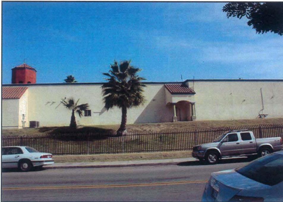
SITE PRIOR TO INSTALLATION
