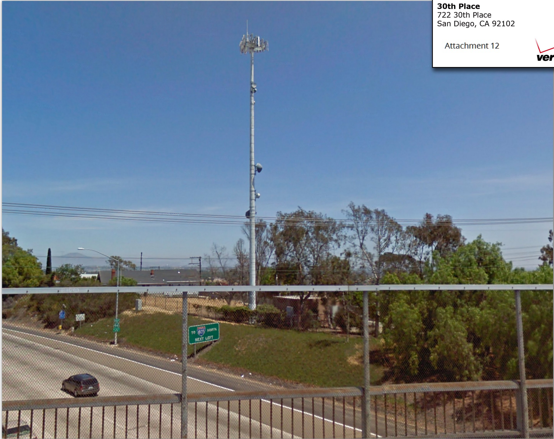
Existing telecommunications site
