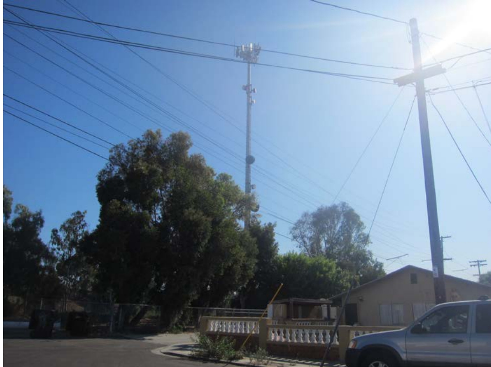
Looking at west elevation
