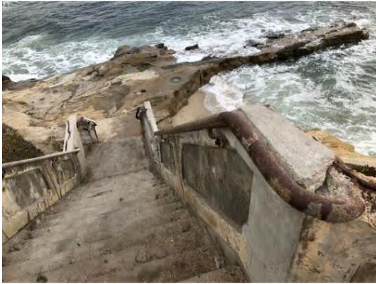
A closer look of the vertical side rails of the staircase, which seem to display initial signs of corrosion.
