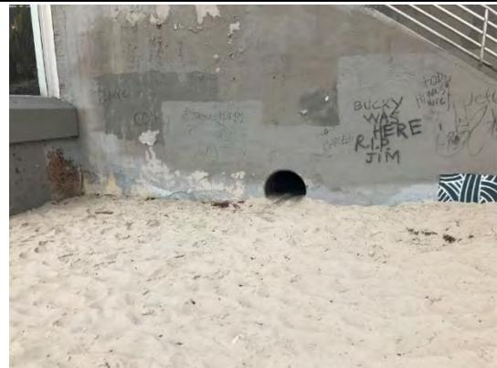
A close-up of a circular storm drain pipe opening in a concrete wall. The area around the pipe is heavily eroded, and there is a significant amount of sand piled up next to it. Graffiti is visible on the wall above the pipe. | <p>The increased sand level next to the storm drain pipe poses a cause for concern.</p>                                             |
