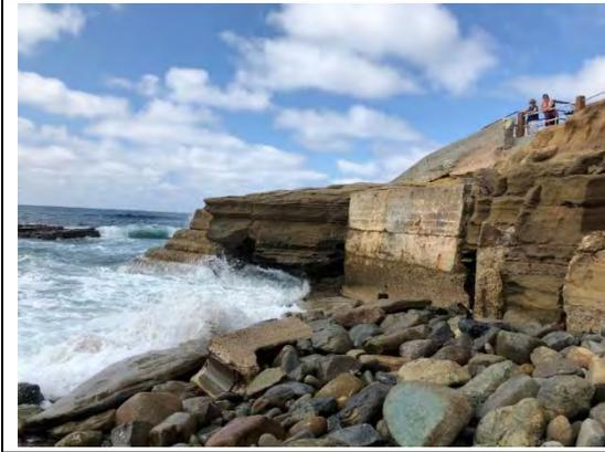
The photograph suggests enhanced erosion on the northern end of the bluff. The pedestrian access way is several feet from the edge of the bluff.
