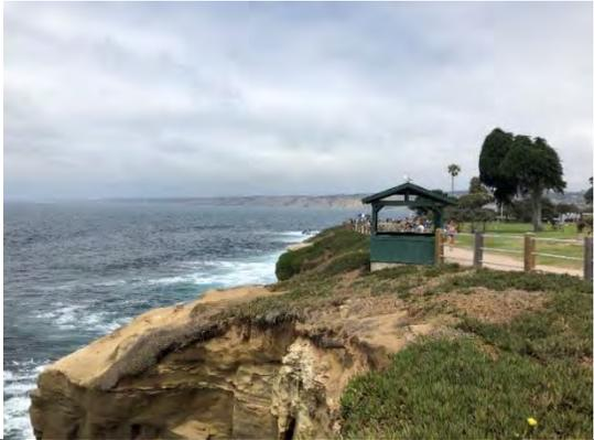
A photograph showing a coastal bluff with a green-roofed lookout structure. The bluff edge is eroded, and there is a gap between the edge and the structure. The ocean is visible in the background under a cloudy sky. | <p>The edge of the bluff suggests that there is marine and subaerial erosion. The photograph also displays the roughly 5 feet between the edge of the bluff and the lookout structure.</p>              |
