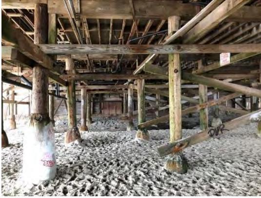
The wooden reinforcement structures underneath Crystal Pier that support the Hotel stay above.
