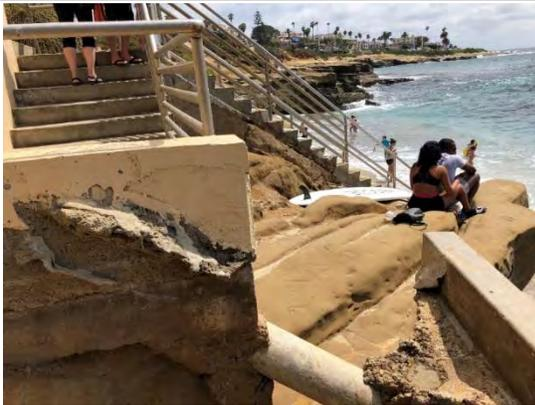
A closer look at the pump next to the staircase. The rock formations around and near the pipe appear to have eroded away. The fractures in the rocks next to the pipe suggest enhanced erosion.
