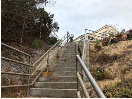
A close-up image of the pedestrian access way. There seems to be slight rusting and cracks within the concrete of the stairs.
