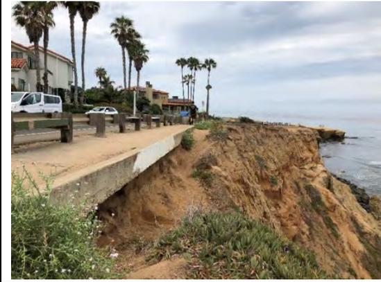
The erosion appears to be approaching the pavement edge in between Hill and Guizot Street.
