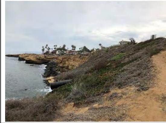
The double-barrel CMP storm drain appears to have not changed. The reconstruction of the slope around the double-barrel CMP storm drain seems to have not changed much since 2003.
