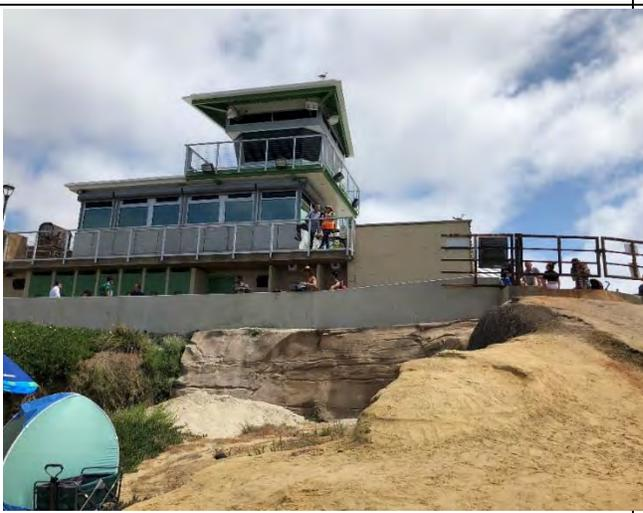
The lifeguard station by Children's Beach appears to be supported along a bluff that experiences marine and subaerial erosion. There appear to be cracks in the Point Loma formation layer underneath the lifeguard station.
