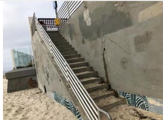
A close-up view of a concrete staircase with metal railings. The wall to the right of the stairs shows a small, dark circular opening (a drain hole) and a vertical crack in the concrete.                                        | <p>A closer look at the staircase; there appears to be a tiny fracture by the drain hole for groundwater.</p>                       |
