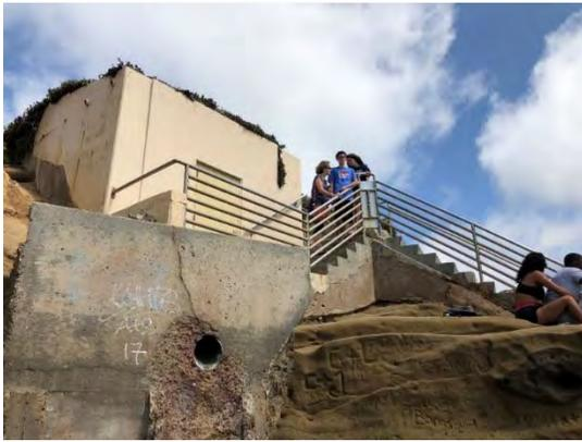
A photograph of the staircase pedestrian access way next to a pump station. The area adjacent to crucial joints of the staircase displays several fractures.
