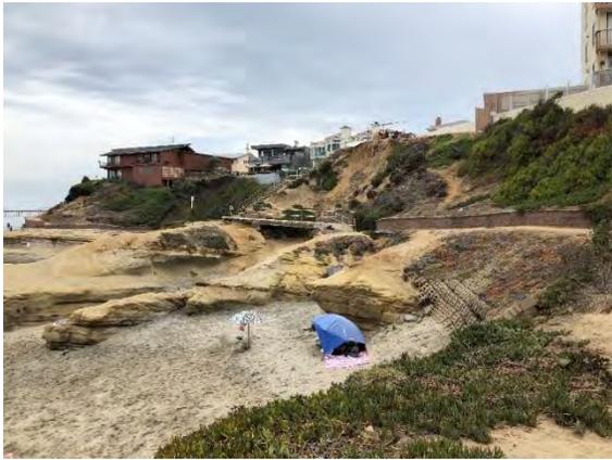
A photograph of a coastal bluff. The bluff is supported by brick structures. A blue tarp is visible on the ground in the foreground. The bluff shows signs of erosion and is partially covered with vegetation. Houses are visible on the top of the bluff. | <p>The brick bluff support structures to the right center side of the photograph appear to be sloped outward at the bottom more so than the two rows above.</p> |
