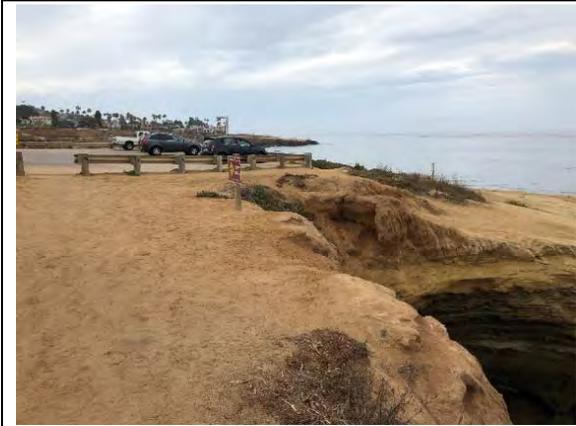
The photograph was taken near the south end of the bluff-top surface and shows how the erosion appears to be approaching the road barrier and pedestrian warning sign.
