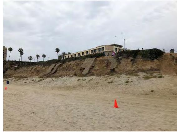
A photograph of a bluff face adjacent to Crystal Pier that contains several reinforcement structures. The bluff face displays signs of marine and subaerial erosion.
