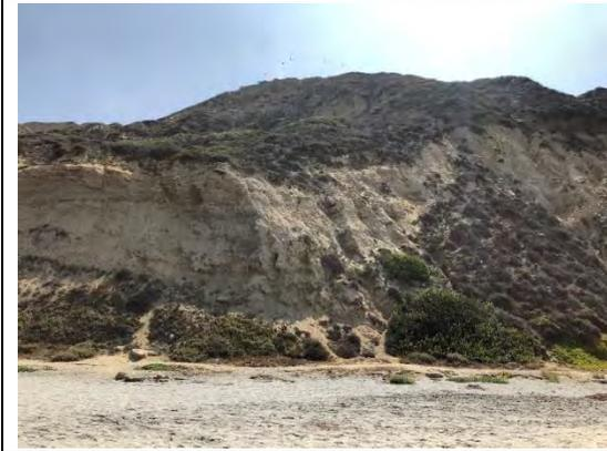
The bluff adjacent to the staircase access from the Gliderport stairs. The photograph suggests marine and subaerial erosion at this point. However, the vegetation on the bluff appears to be supporting the structure.
