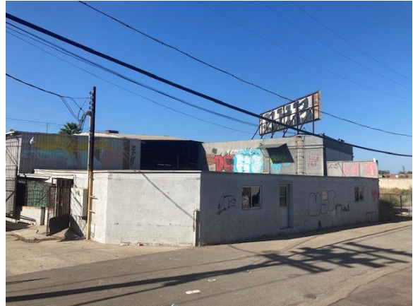
Picture 2 - Westerly view from alley
