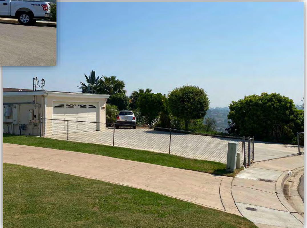
Photo 2. View from the Southwest
