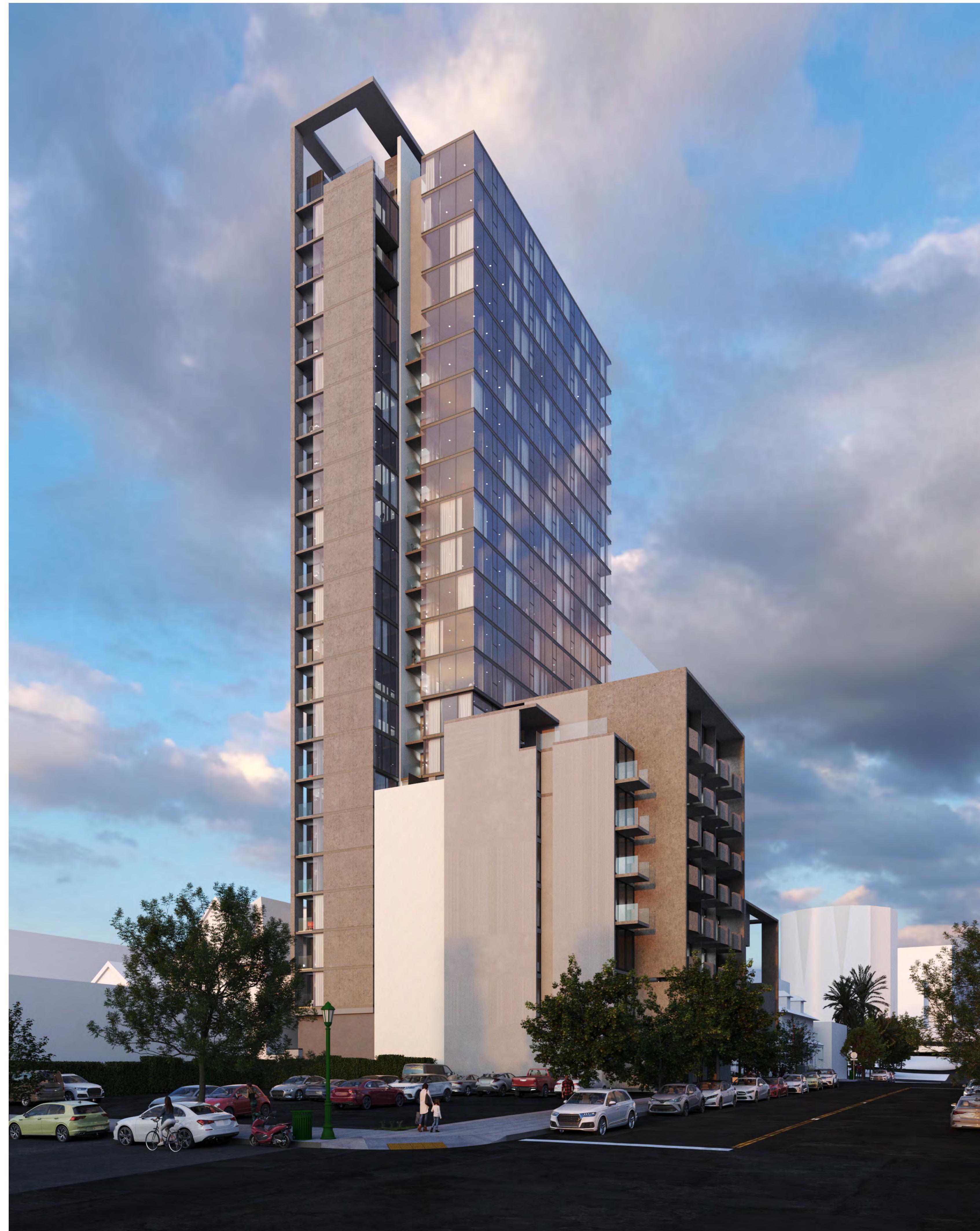
VIEW FROM WEST CEDAR STREET LOOKING EAST
