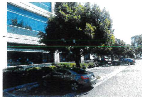
PHOTO 1 LOOKING SOUTHWESTERLY AT BUILDING ZONE ONE
