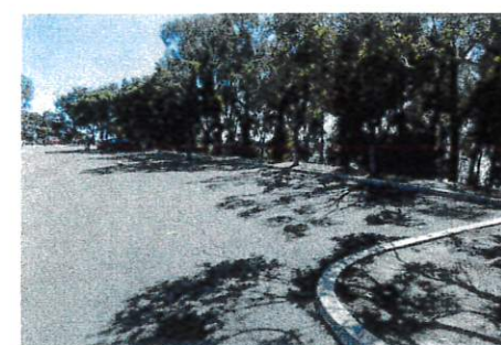
PHOTO 4 LOOKING WESTERLY IN ZONE ONE
