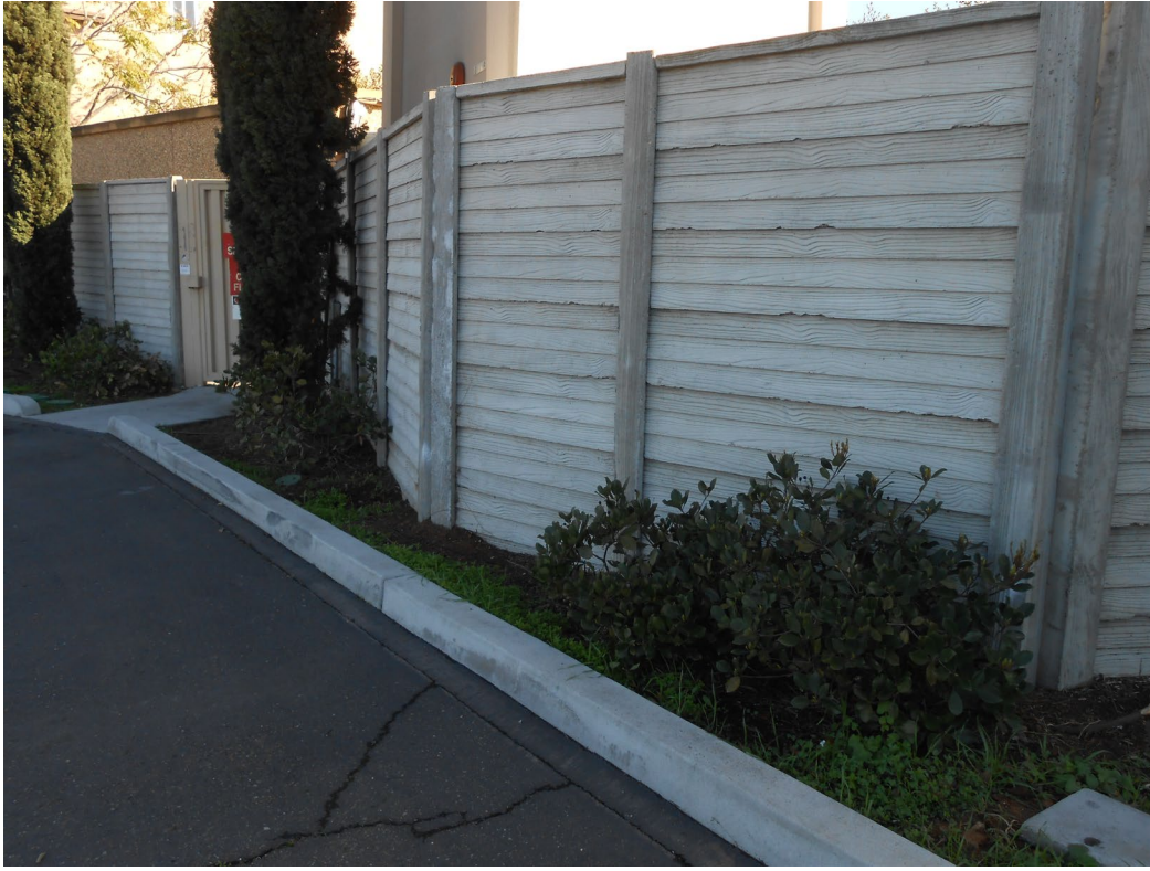
North elevation of the equipment enclosure
