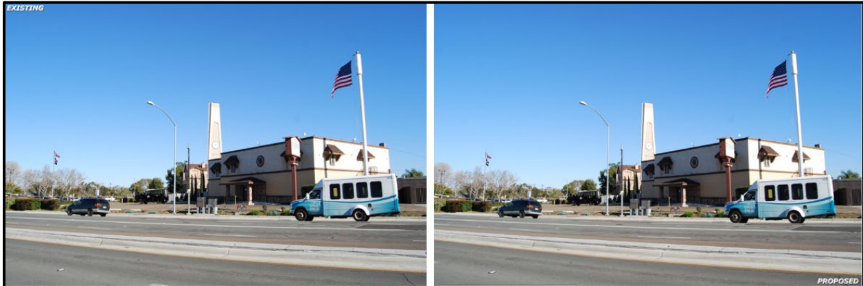
Figure 2: View of WCF tower from Linda Vista Road
