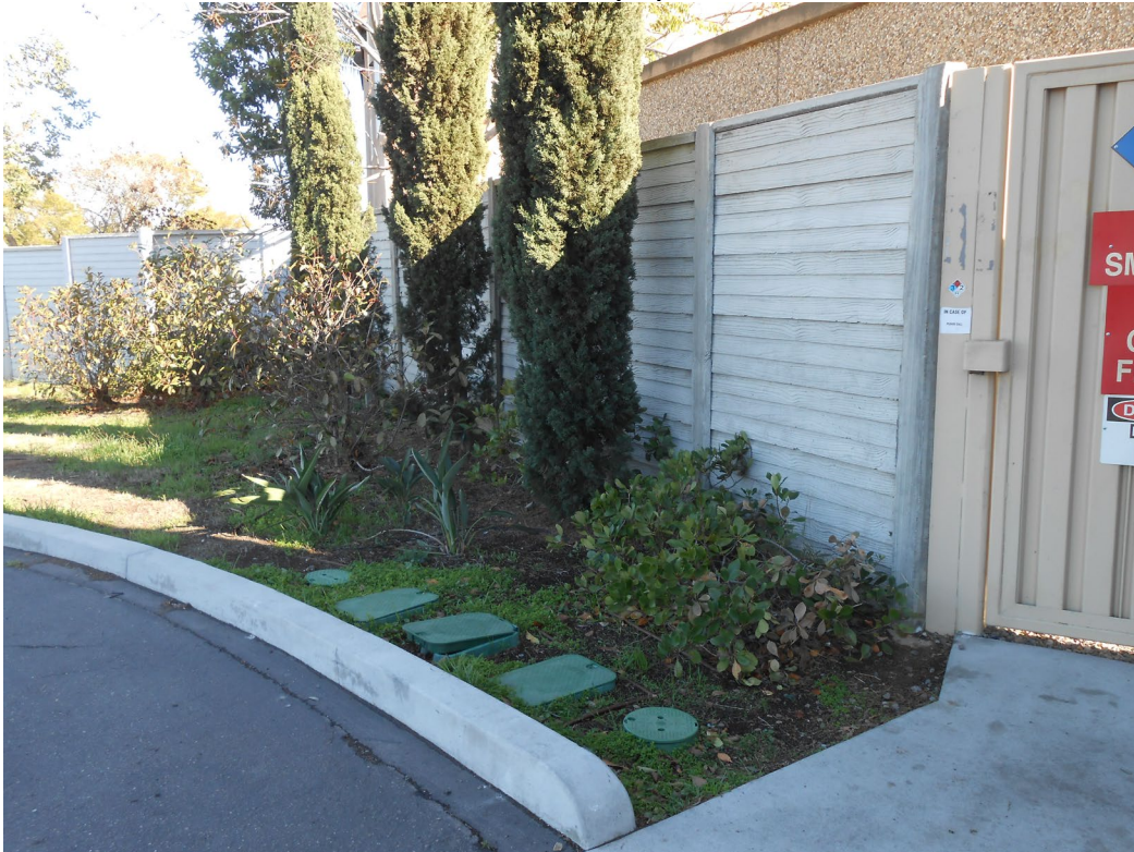
North elevation of the equipment enclosure
