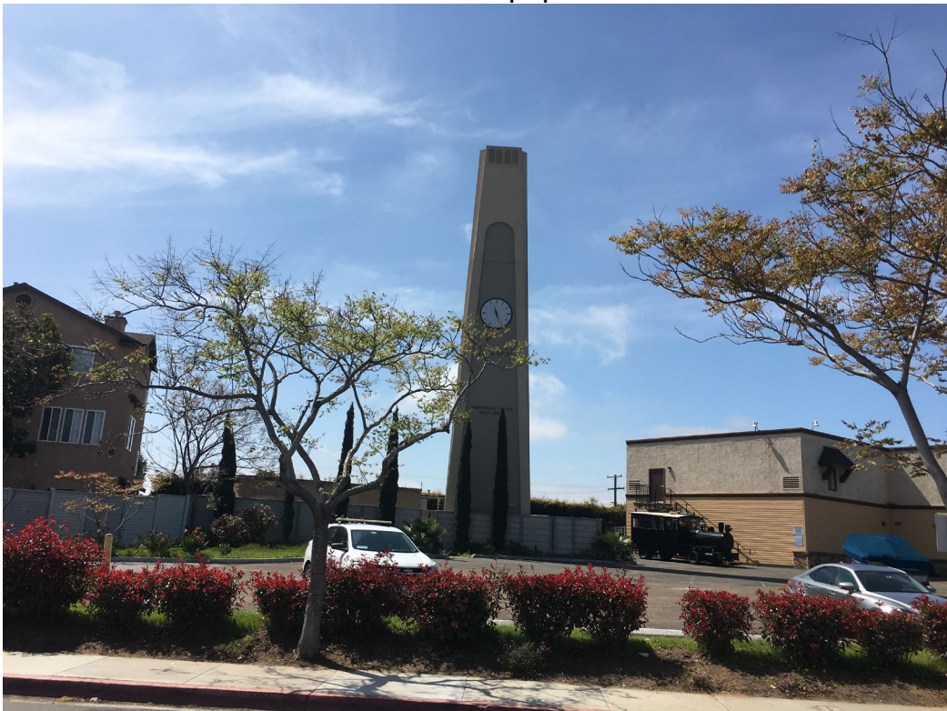
North elevation with equipment enclosure visible at base of tower
