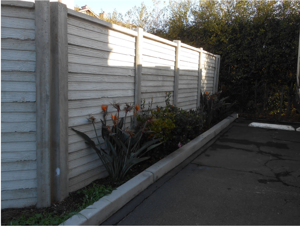
West elevation of the equipment enclosure
