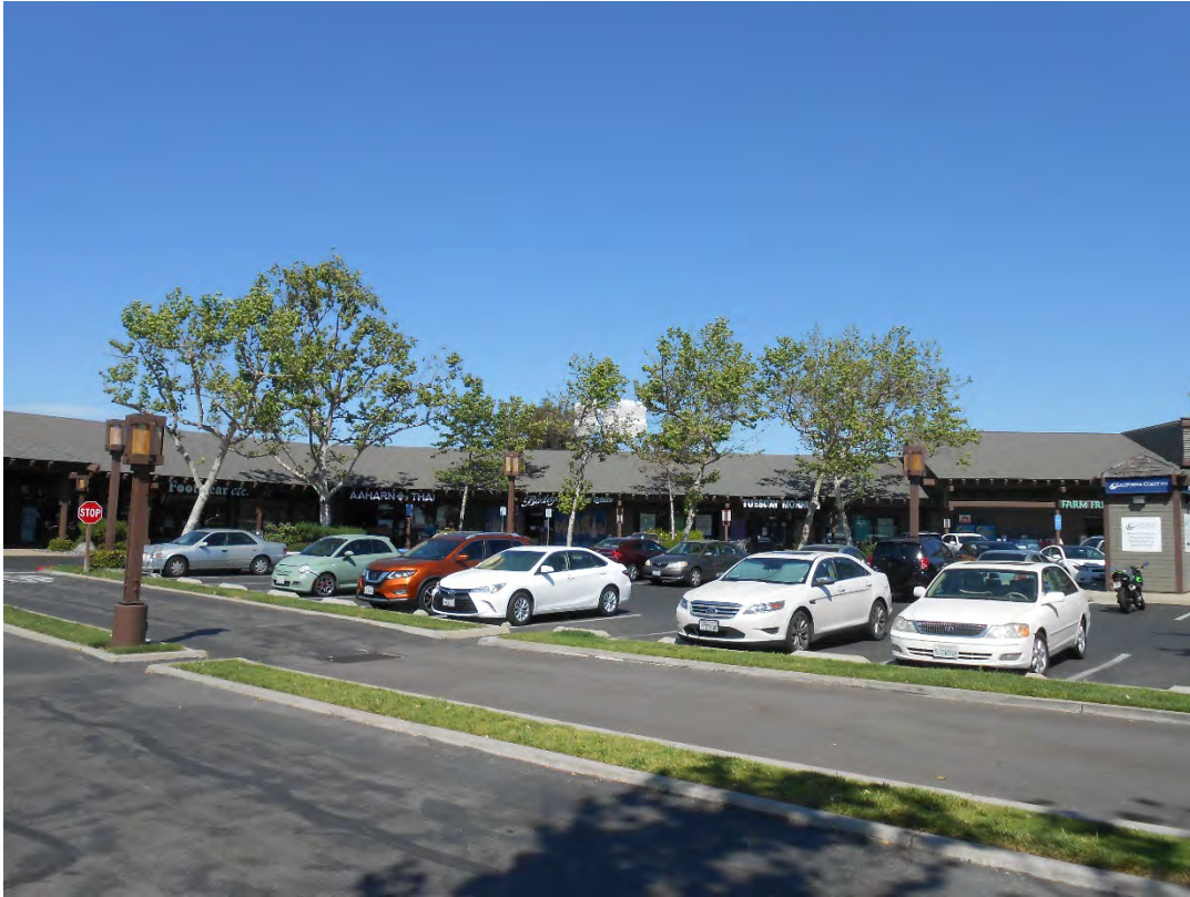
West Elevation – Photo 1
