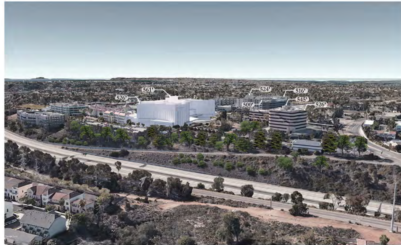
2 PHOTO - FROM I-805 (LOOKING WEST) 1:125
