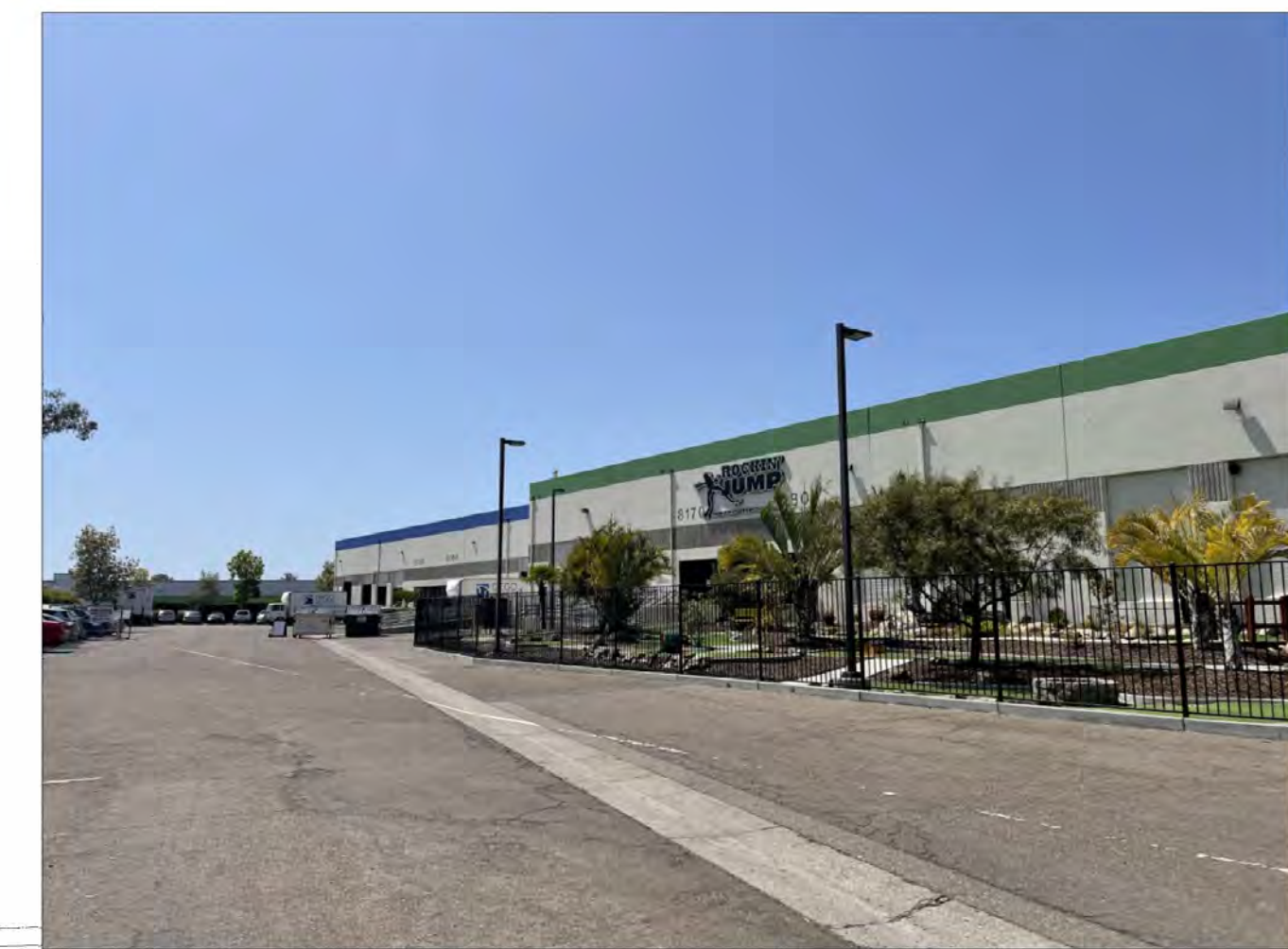
STREET VIEW PHOTO HH
