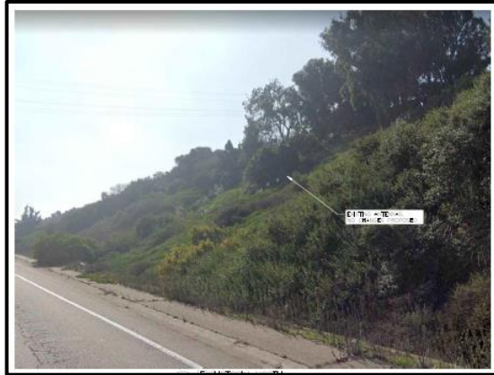
Figure 2: Southerly view of existing WCF monoshrub from La Jolla Parkway
