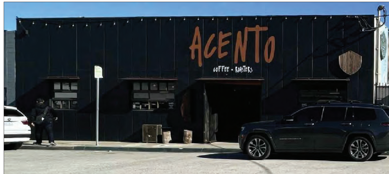
7. Image of Existing West Elevation
