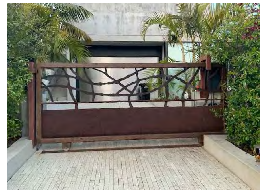
EXISTING IMAGE OF THE SILVERADO ST. ROLLING GATE INDICATING THE TOP 3' AS A 75% 'OPEN FENCE' AS PER SECTION 142.0310(c)(3)(A) OF THE SDMC.
