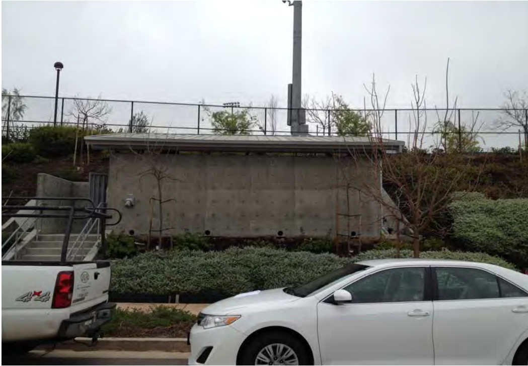
VIEW NO 6. LOOKING SOUTHEAST FROM NIGHTHAWK LANE OF EQUIPMENT ENCLOSURE
