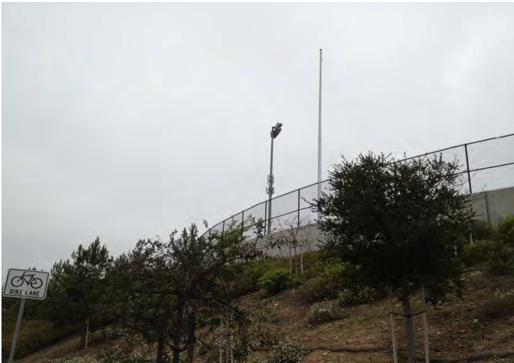
VIEW NO. 3 LOOKING NORTH FROM CAMINO SAN BERNARDO
