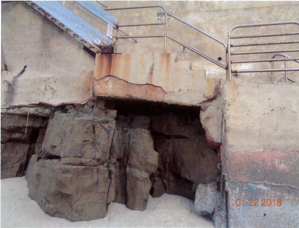
Foundation of stairway now unsupported
