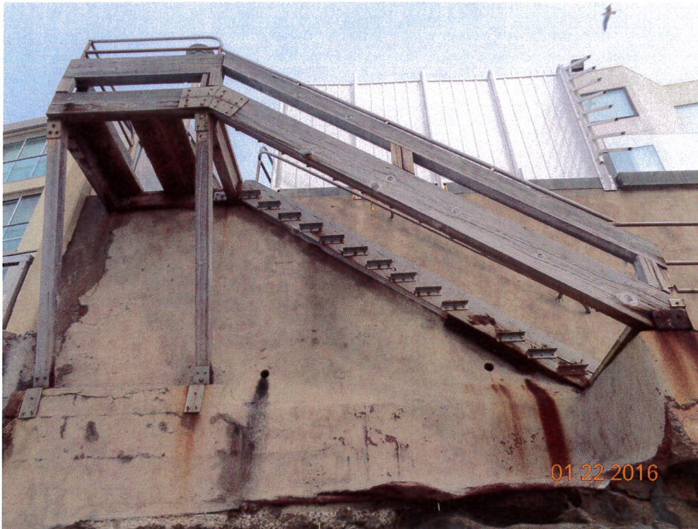
Remains of wooden stairway after storms. Wood has since been removed and the access point barricaded.
