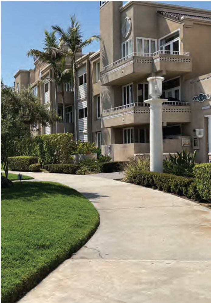
Accessible, interconnected pedestrian routes improve walkability.
