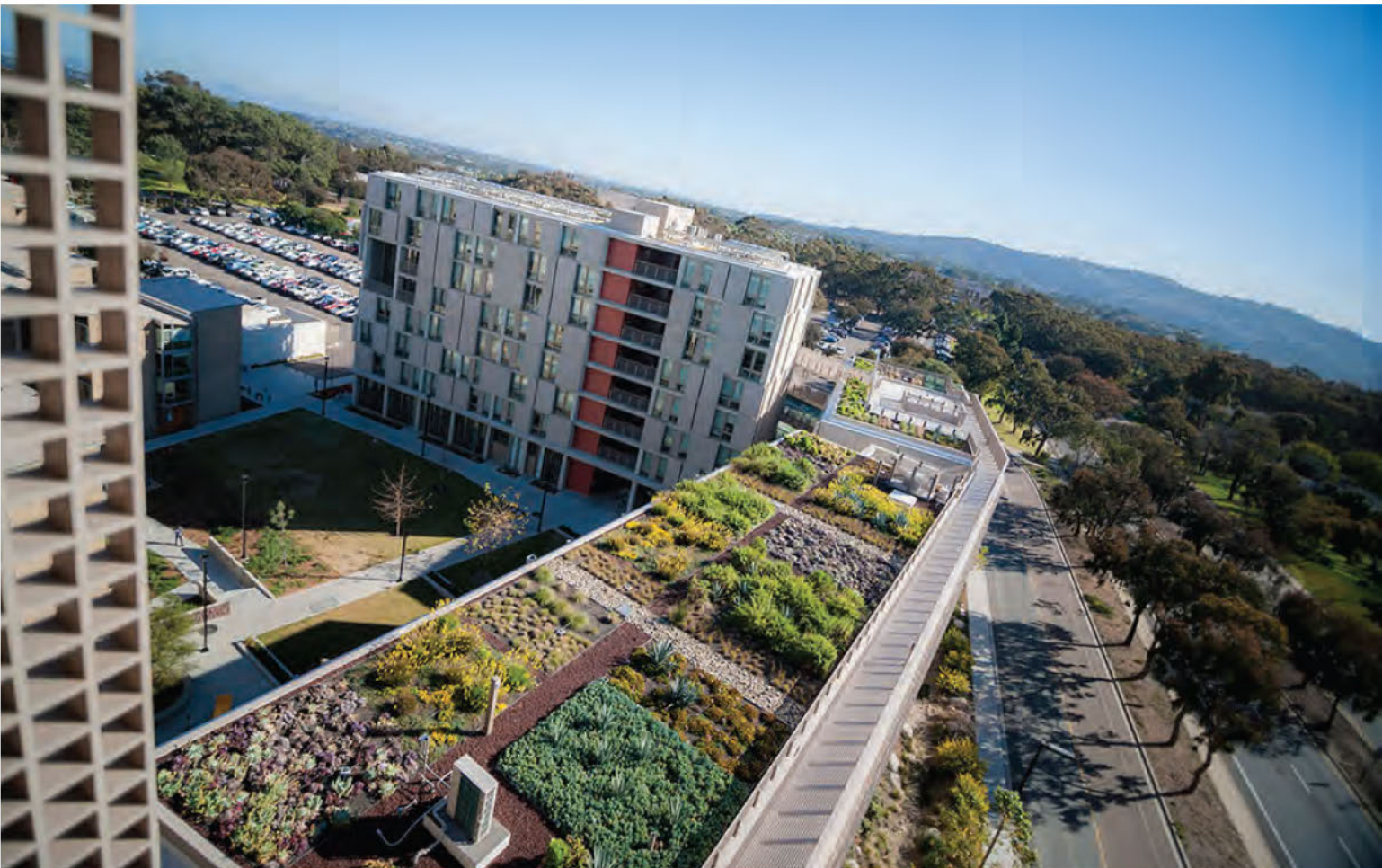
Green roof implemented at the Keeling Apartments. - Source: UC San Diego Publications
