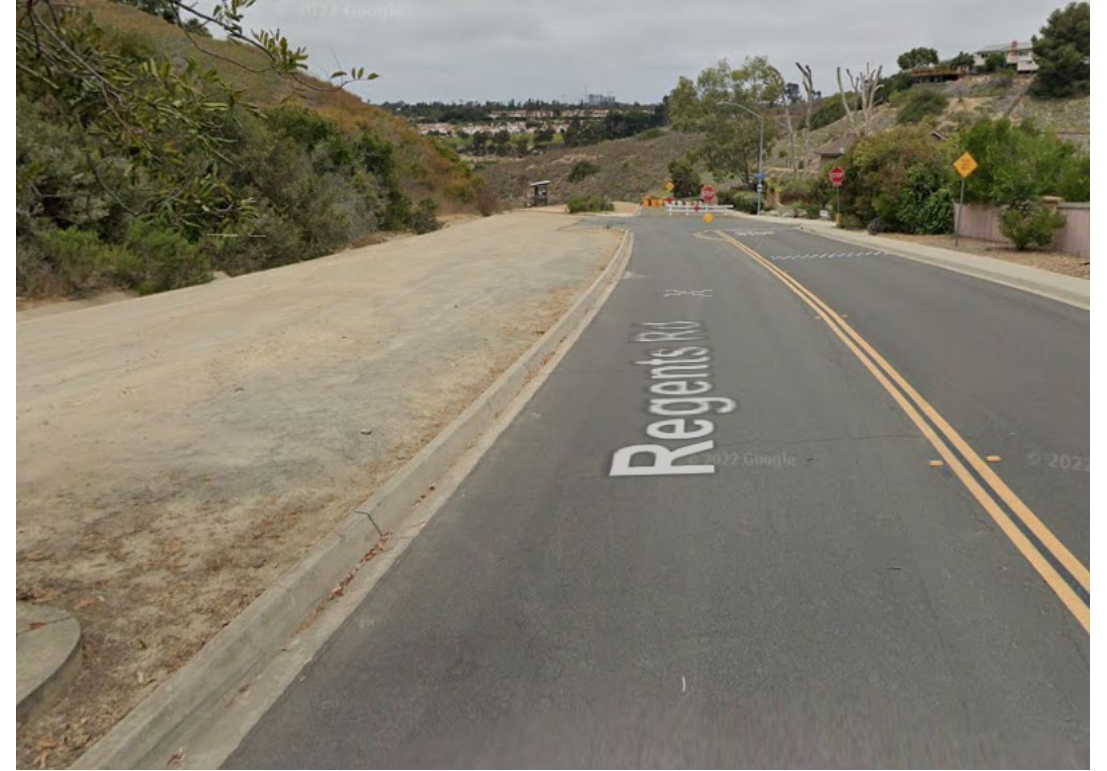
Existing Conditions at Regents Road South Taken on Google Street View 2023
