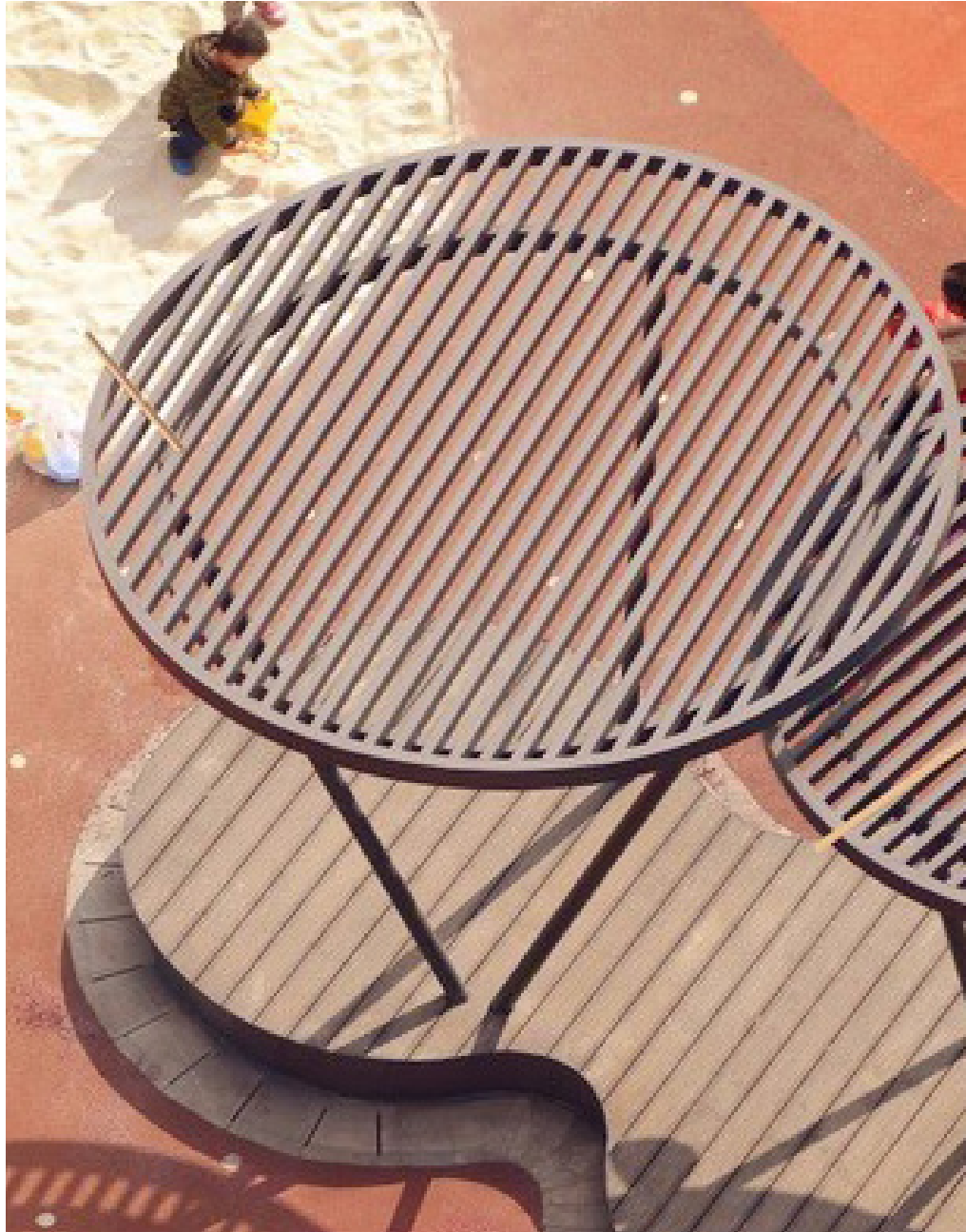
ROUND SHADE STRUCTURE WITH METAL SLATS
