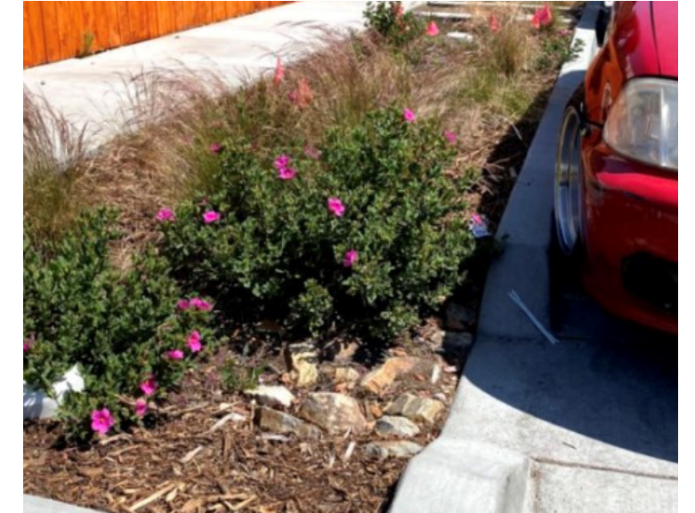
GREEN GUTTER PLANTER Curb Cut
