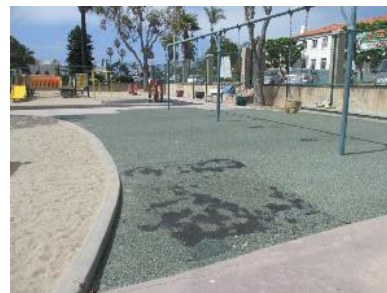
Playground surfacing in need of repairs
