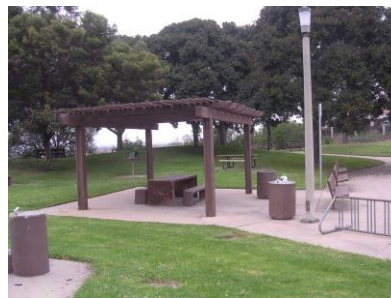
Site furnishings need replacement
