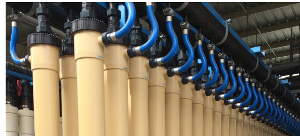
Barrier 3 Membrane Filtration
