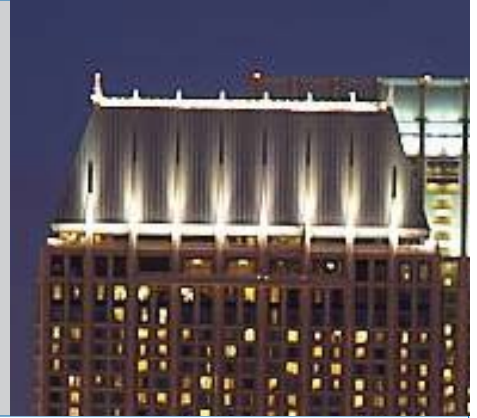
Photo 3.40: Lighting can emphasize the complex structural system of a roof design.
