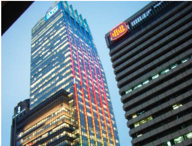
Photo 3.63: LED light sources can be integrated into architectural features of a building.
