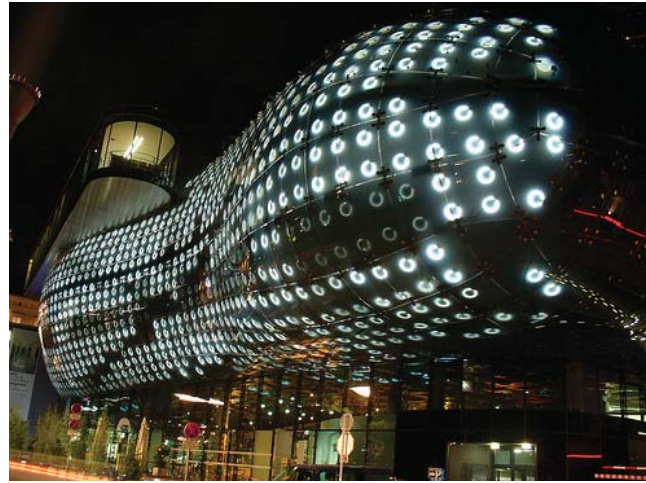
Photo 3.54: Lighting can add to the unexpected variations in the fine grain of the streetwall. Rings of light are embedded in the exterior skin with controllable illumination levels. Kunsthaus Graz Museum, Austria.
