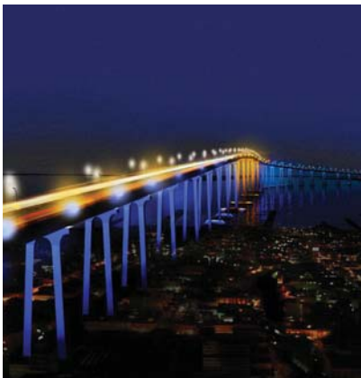
Photo 3.19: Programmable LED light treatments along the Coronado Bridge. Peter Fink (Form) proposal for the Coronado Bridge. Dynamic lighting offers flexibility to define arrival threshold to identify surrounding areas from a distance.
