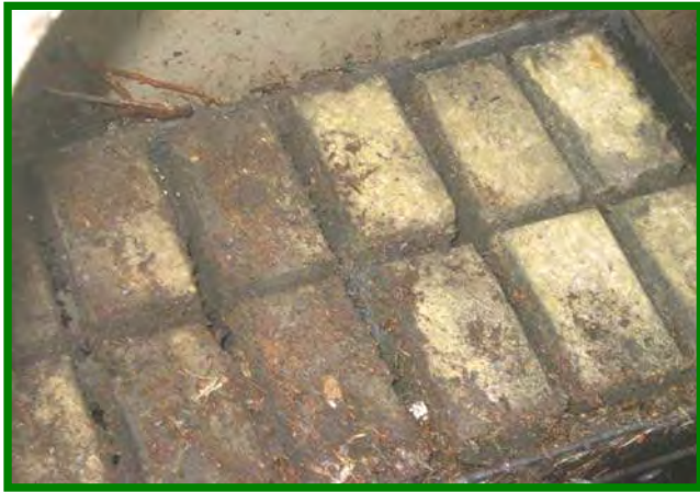
Remove Spent BioMediaGREEN Filter Blocks
