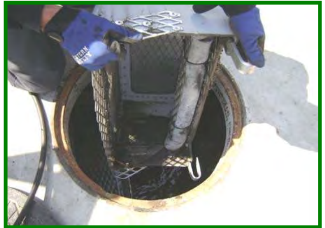
Remove Catch Basin Filter
