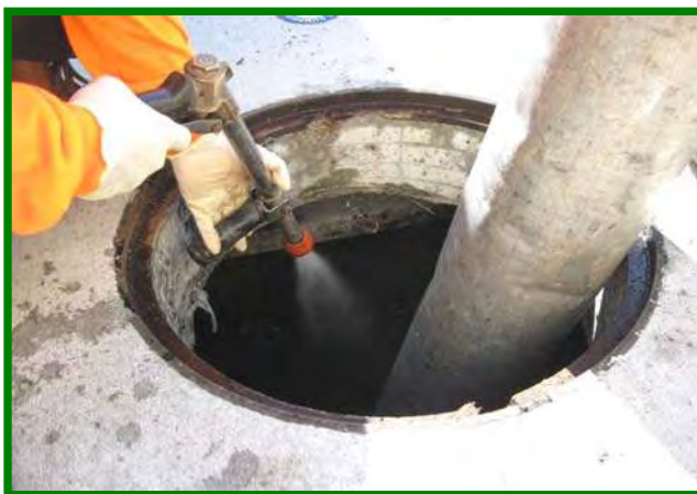
Vacuum out the Sediment Chamber
