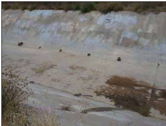
Figure 2-1. SD8(1) Mass Loading Station
