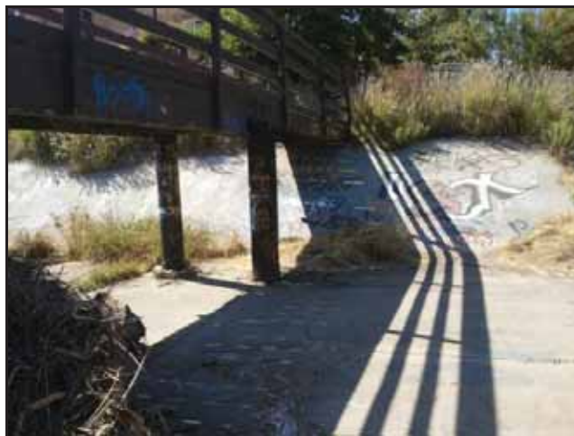
Figure 2-2. DPR3 Mass Loading Station
