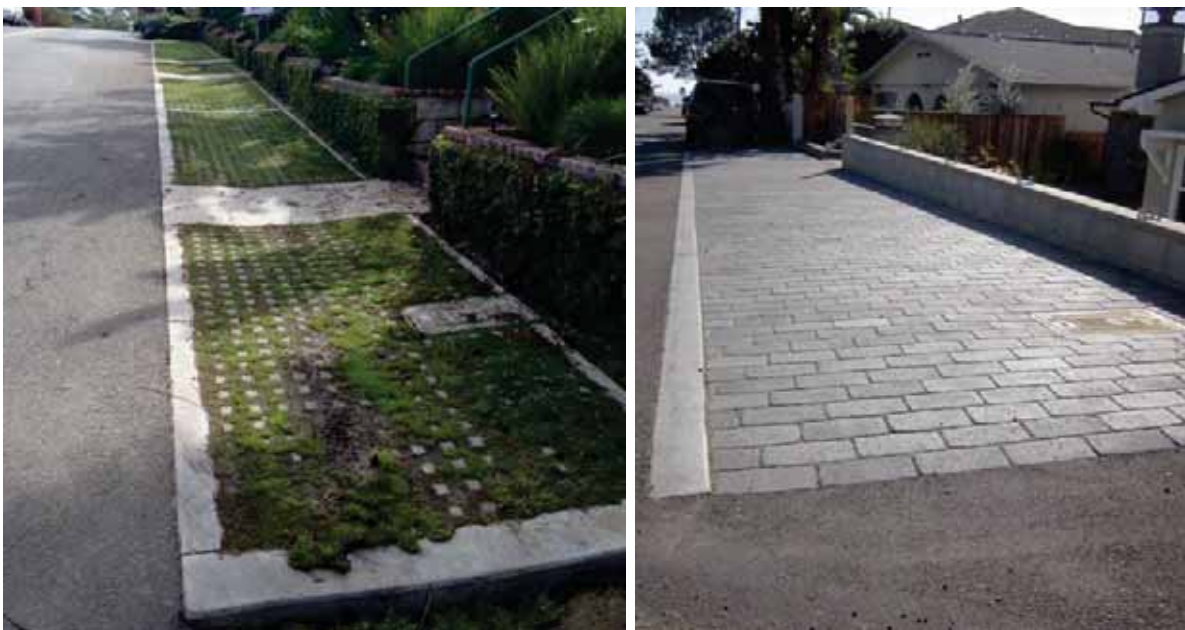
Figure 4-8 Permeable Pavers in the Right-of-Way Without Curb and Gutter
