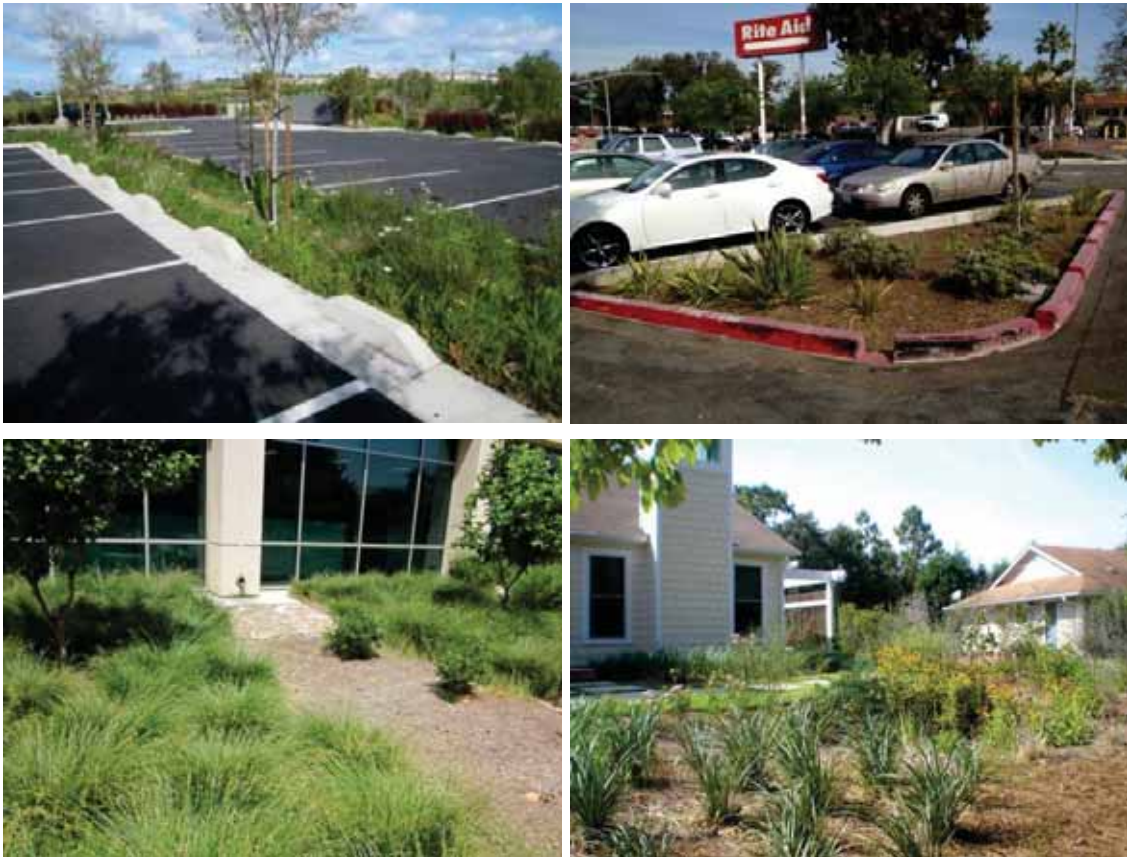
Figure 4-5 Bioretention Areas in Parking Lots and Adjacent to Buildings Provide Multiple Benefits by Treating Runoff While Also Serving as Landscape Features and Habitat
