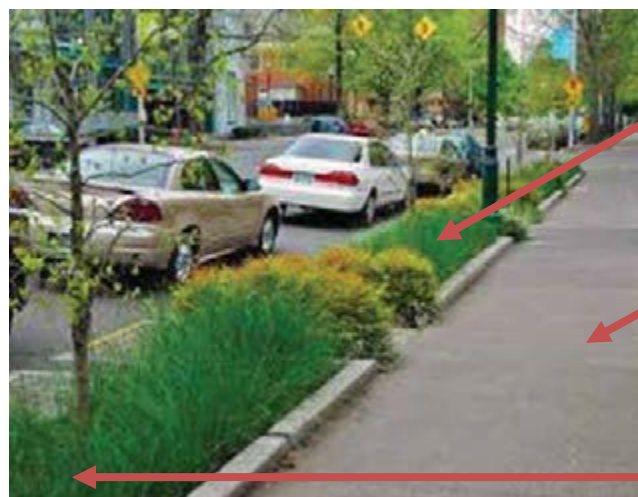
Figure 1: Illustration of Sample Structural BMP: Green Streets
