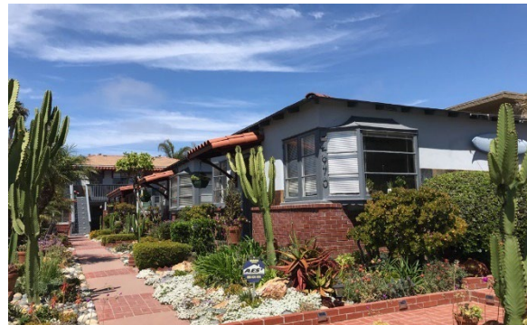
Half bungalow court at 4970 Cape May Avenue with L-shaped plan, detached units, minor variation.
