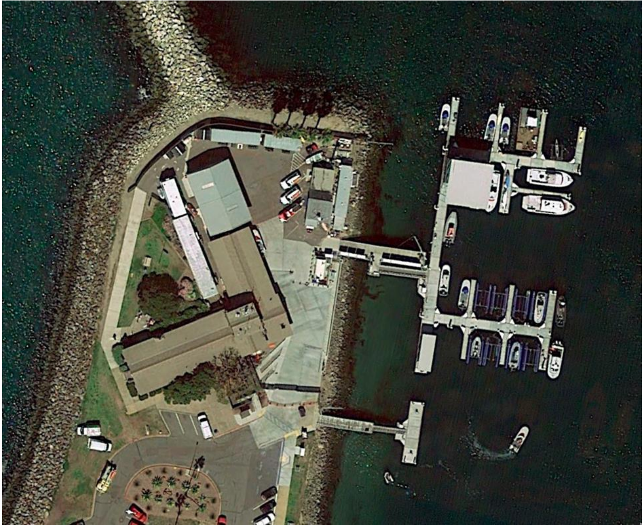
Figure 2—Lifeguard Headquarters Aerial View
