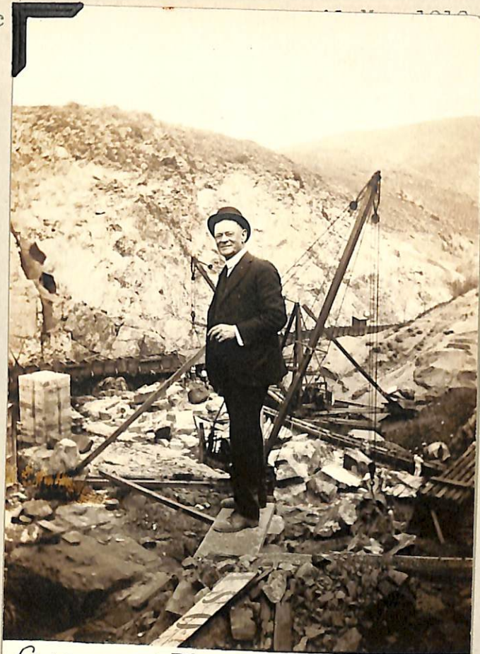
COUNCILMAN THOS. J. FISHER at Lower Otay Dam - Aug. 1918.
