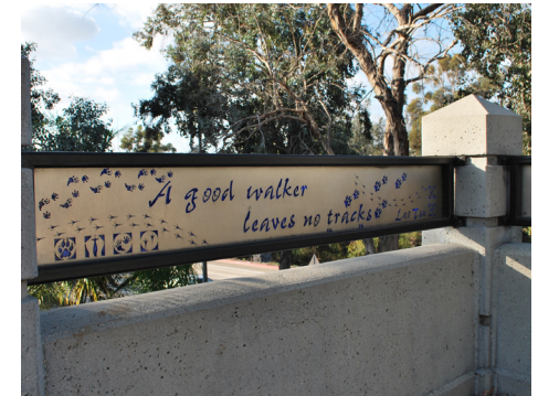
Public art incorporated into bridge railing.
