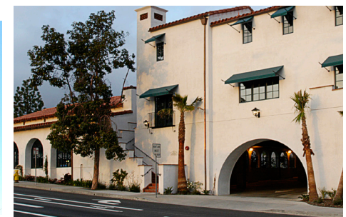
Examples of residential development with parking structures.
