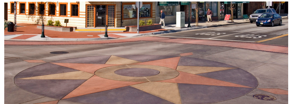
Crosswalk striping and intersection specialty paving enhance the area and distinguish the pedestrian realm from vehicular areas.
