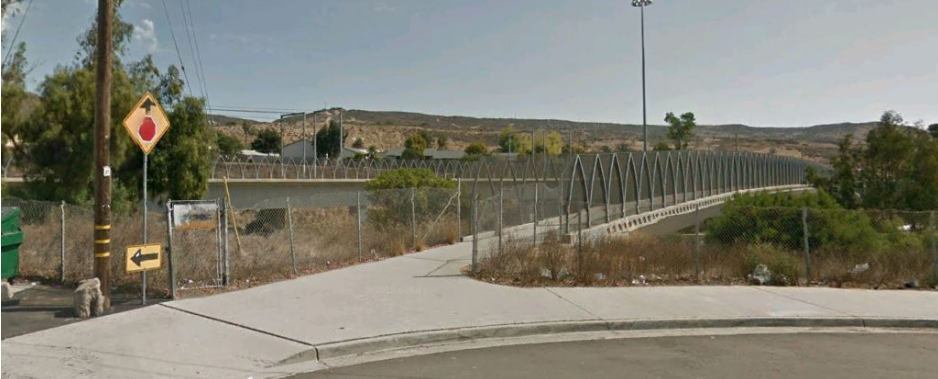
Existing condition at Olive Drive
