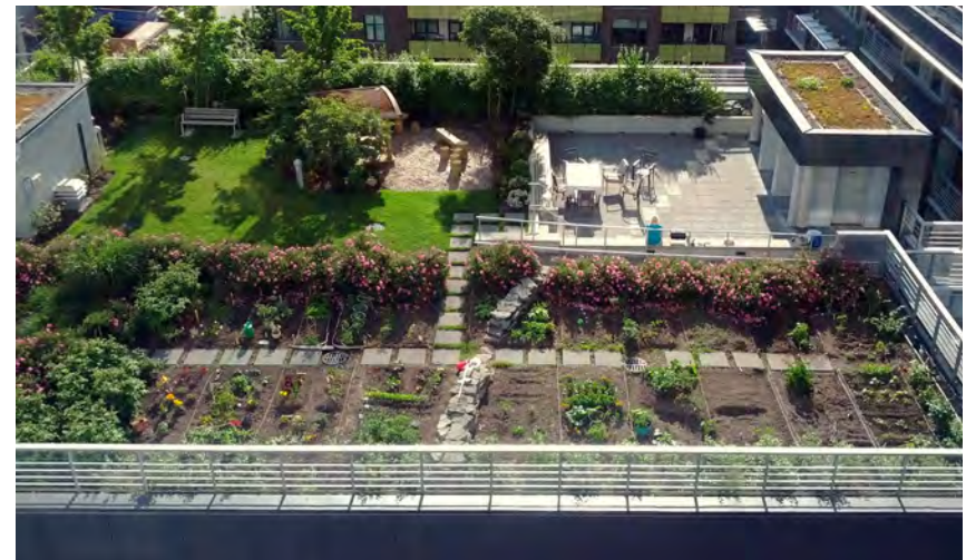
There are many creative ways to increase energy and water efficiency and climate resilience, including green roofs and rooftop gardens.
