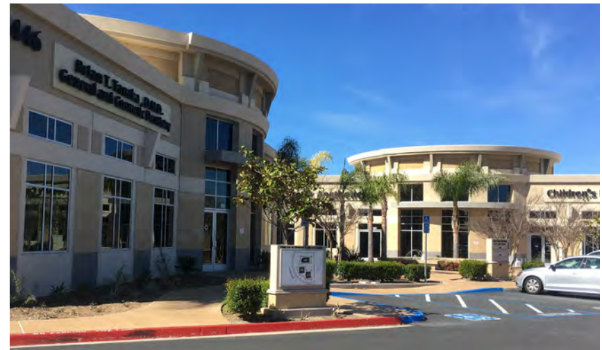
Health care and human services facilities in Midway - Pacific Highway provide services to many San Diegans and can incorporate design elements and operational activities that ensure compatibility with the community.
