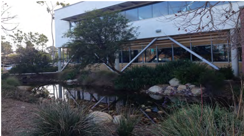
A storm water infiltration bioswale at the West City Continuing Education Center at work.
