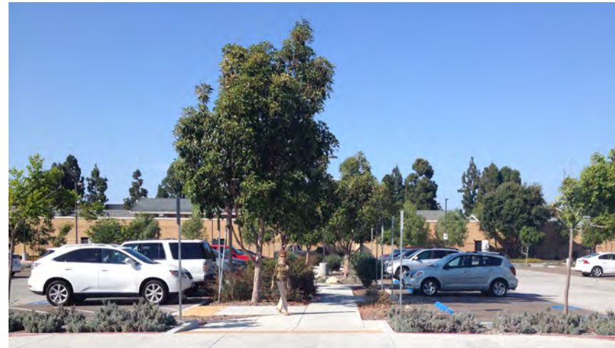
The West City Continuing Education Center is an excellent example of site design for storm water management and features porous concrete and bioswales in its parking lot.
