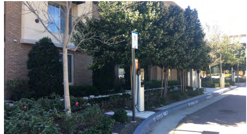
Incorporating emerging technologies such as electric vehicle charging stations as part of infrastructure and development projects will encourage and support sustainable travel choices.
