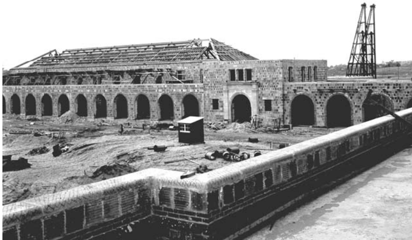
The Marine Corps Recruit Depot under construction.
