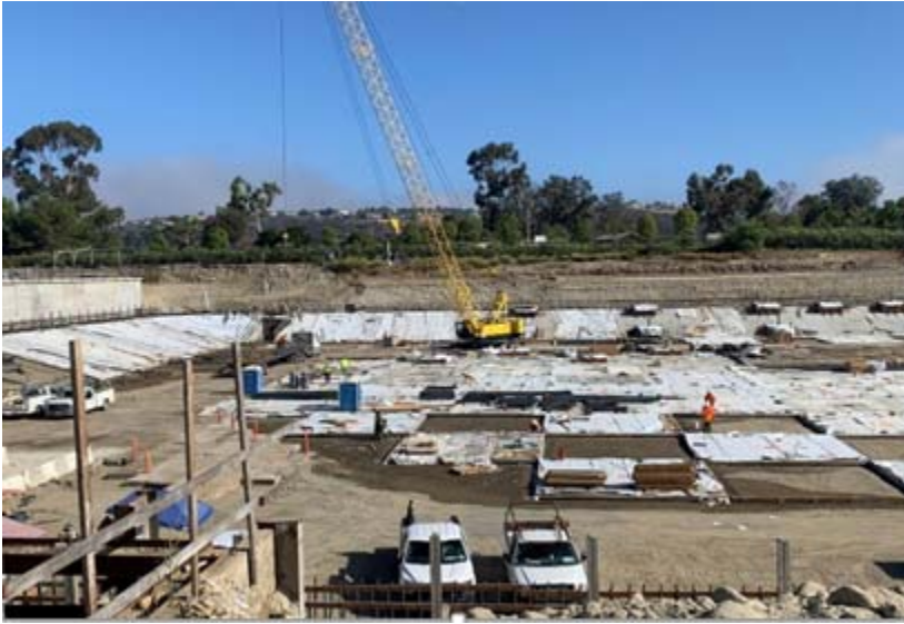
Clear well 1 slab fabrication
