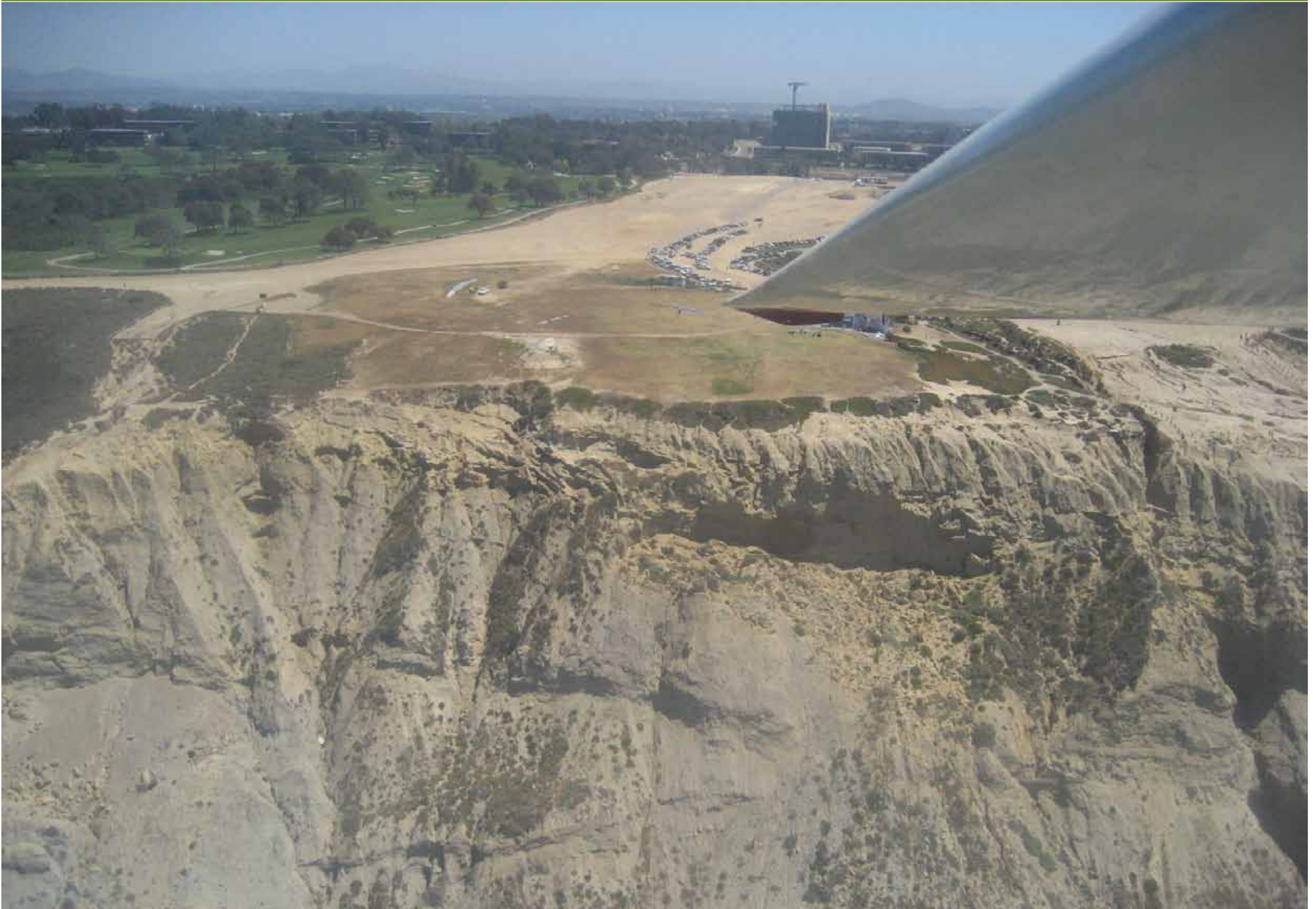
Airfield – Existing Condition
