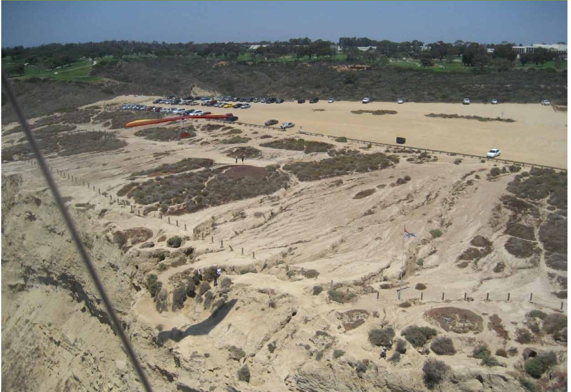
North Bluff – Existing Condition
