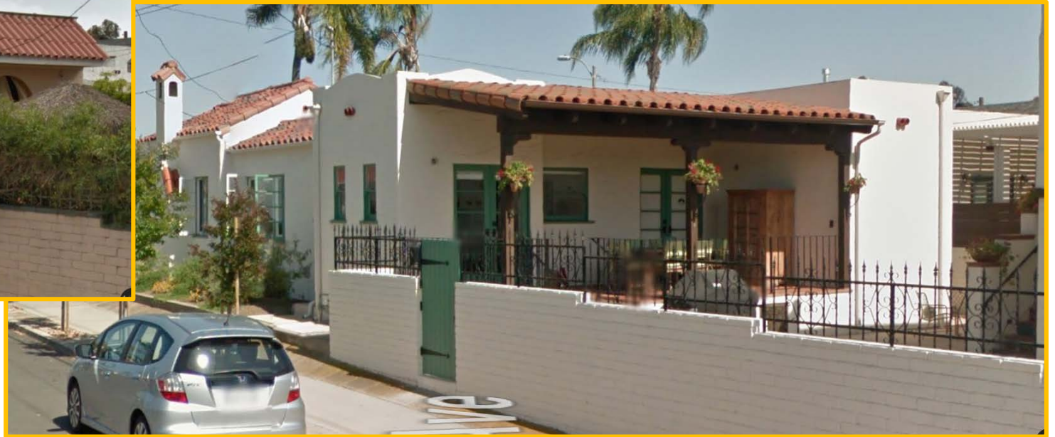
HRB Site #1008-061, 3448 Pershing Avenue: Removal & Replacement of Rear Porch Addn & New Rear Addn
