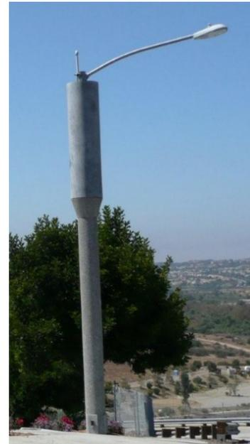
*Figure 26: Macro (non-small cell) right-of-way site with antenna shroud*
