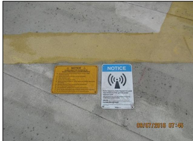
Figure 8: Place RF protective devices on the flat roof/ ground.
