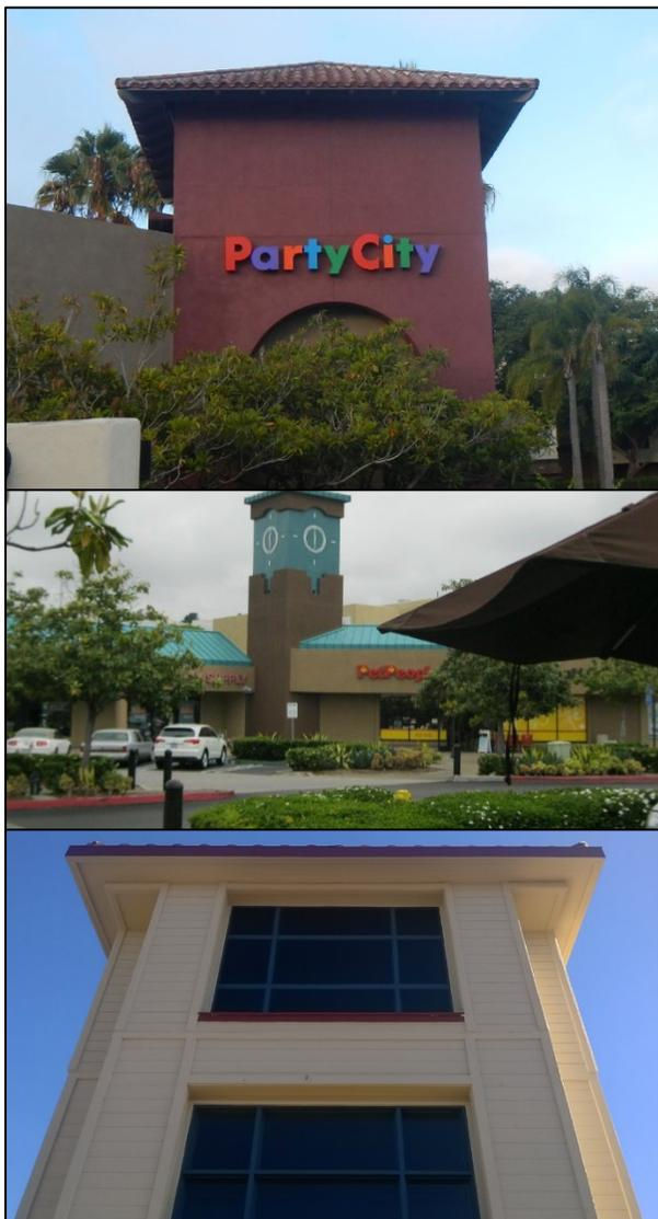
Faux Architectural Elements – Antennas concealed entirely within existing or proposed architectural elements on an existing building. Façade-concealed antennas that present as architectural elements of the building are considered faux architectural elements rather than façade-concealed antennas.
