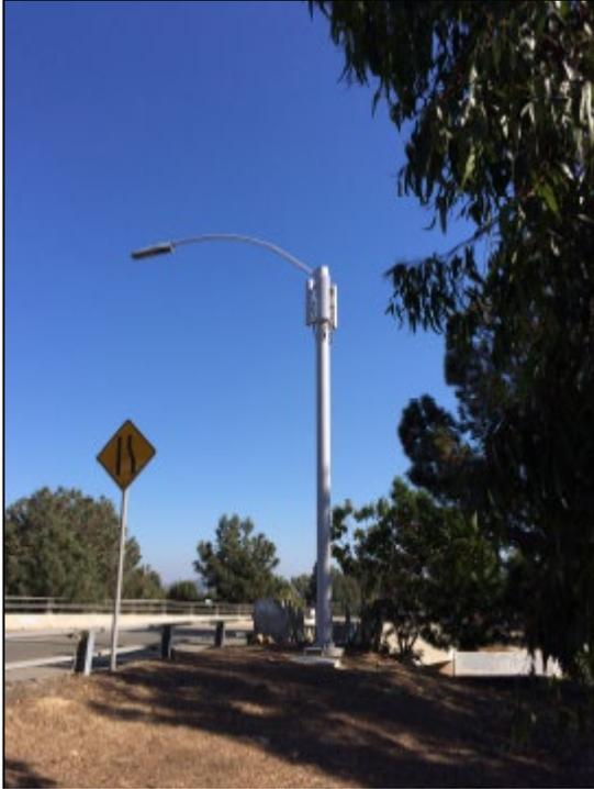
*Figure 27: This right-of-way installation has three antennas mounted flush to the pole with no pipe mounts and no antenna shroud. This is an older installation with no chin covers; they are now required.*
