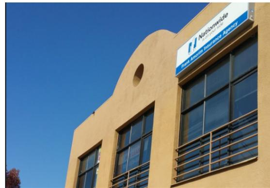
Figure 13: Antennas are concealed behind the circular element.
