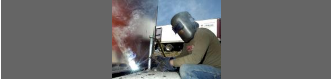
Bret Erickson, of Paso Robles Tank, Inc. & Central Coast Stainless, welds the bottom chime of a big steel water tank being built at the Delta View Golf Course on Thursday, May 8, 2008 in Pittsburg, California.
